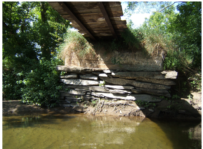
Figure r. Left abutment of recommended bridge replacement project just downstream of M09 reach boundary
