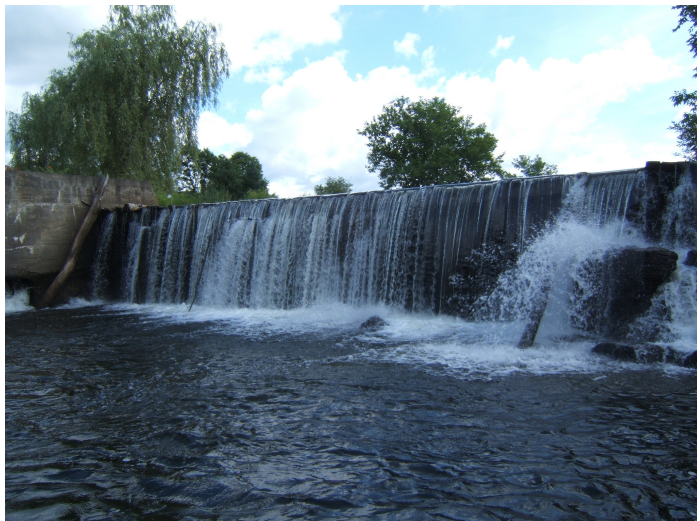
Figure t. Dam/Grade control upstream of Rte 15 crossing
