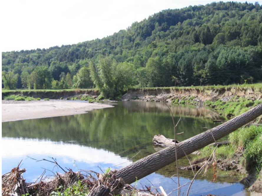
Figure 3: Bank Failure near Longley Bridge Road
