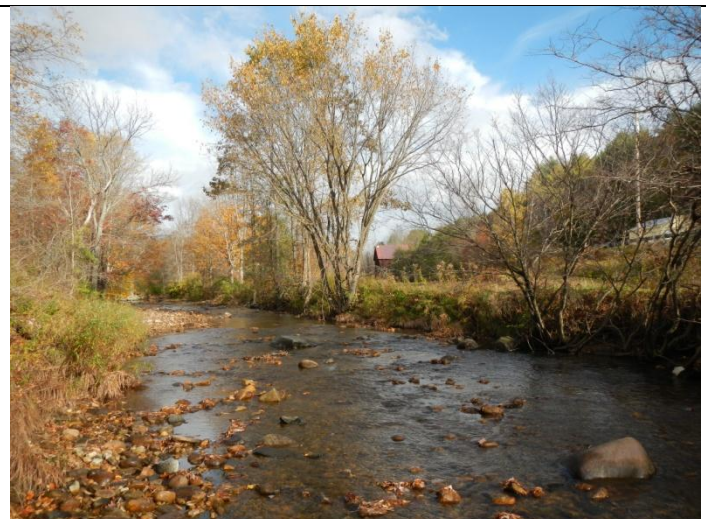
No floodplain benches due to bank scour and armor
