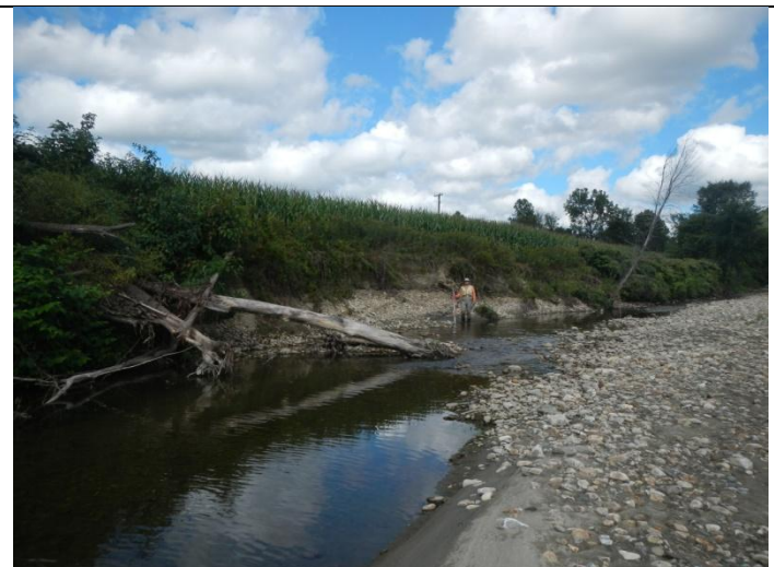
Major bank erosion source of material for deposition
