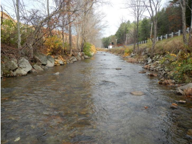
Figure 4.19: Reach M14 straightened along Rt-103.
