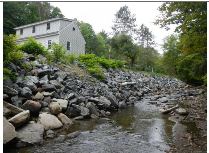
Riprap armor along south bank mid-segment
