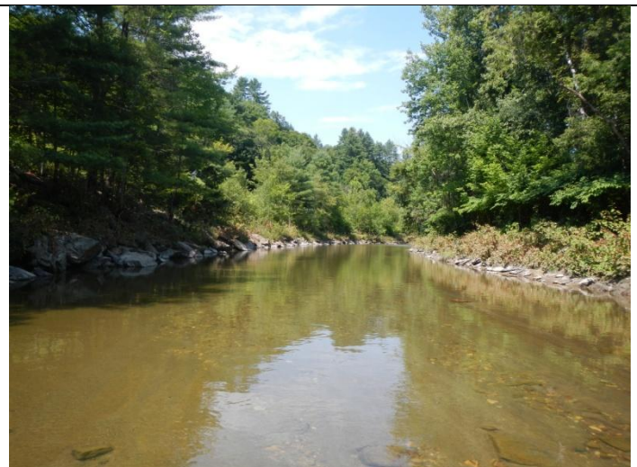
Banks straightened and armored for long sections
