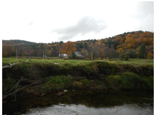
Figure 4.13: Extensive bank erosion along a pasture in reach M14.
