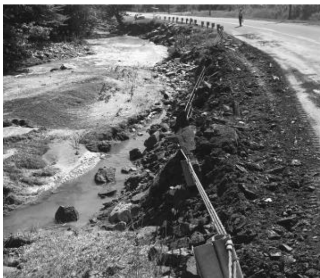
Figure 1.6: Damage from the 1974 flood along the Middle Branch of the Williams River (UVM Landscape, 2011).
