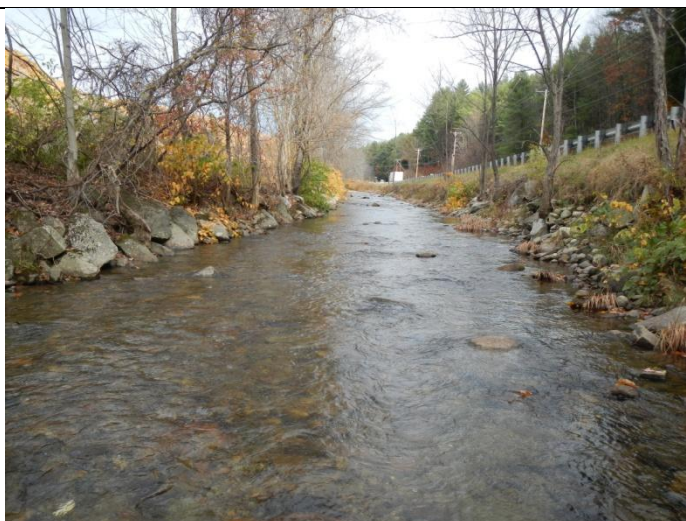
Straightening and bank armor frequent throughout M14
