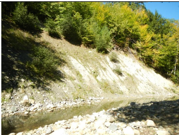
Multiple active mass failures are present in the reach
