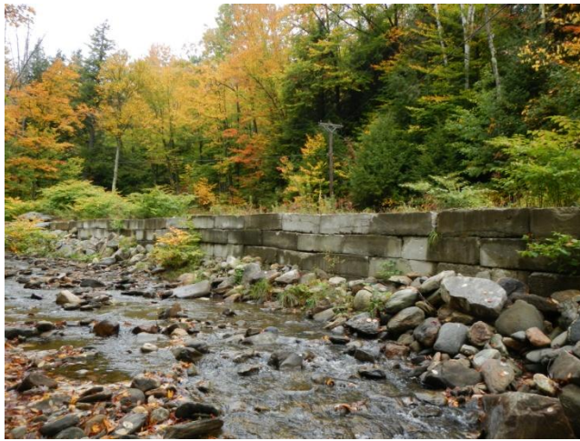
Figure 4.10: Stacked stone wall along Nudist Camp Rd in reach T5.S1.08.
