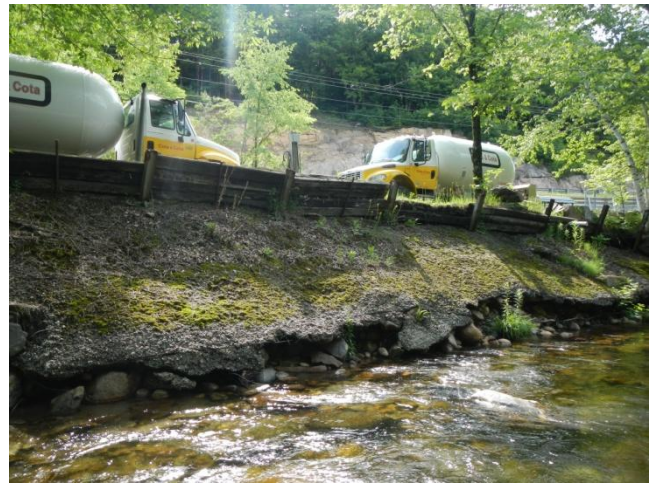
Figure 4.11: Paved left bank along reach M16.
