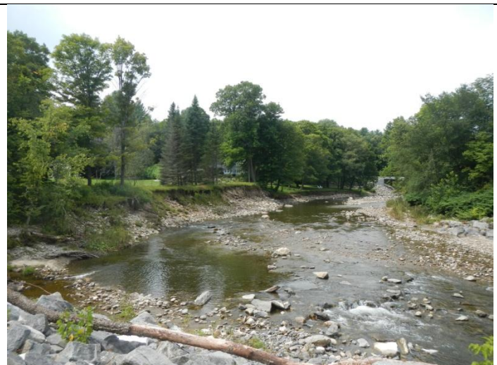
Bank erosion at confluence with tributary
