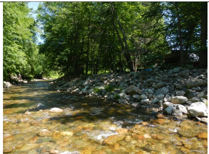
A berm on the right bank protects houses
