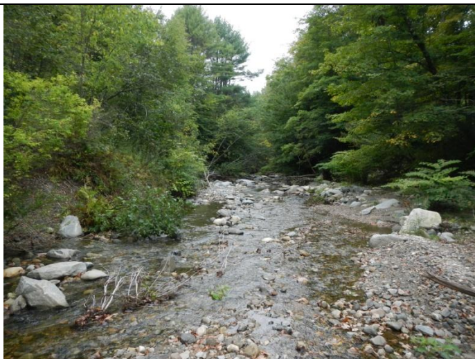
Scouring and widening removed floodplain benches
