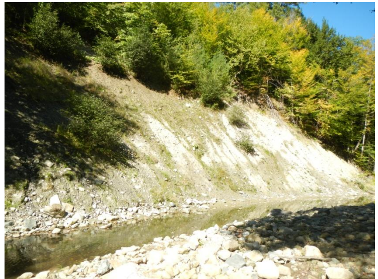
Mass slope failures along Reach T5.06 on the Middle Branch of the Williams River
