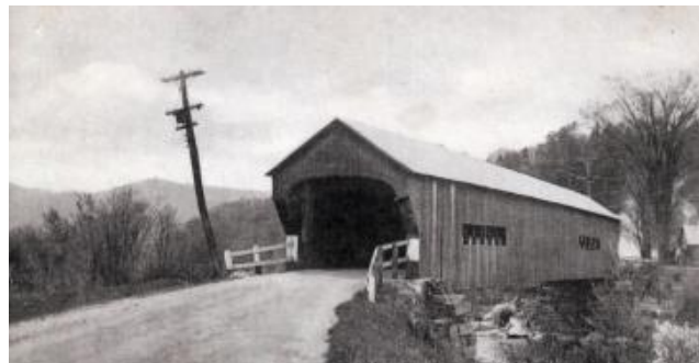
Figure 1.8: Historic photo of the Bartonsville covered bridge (UVM Landscape, 2011).
