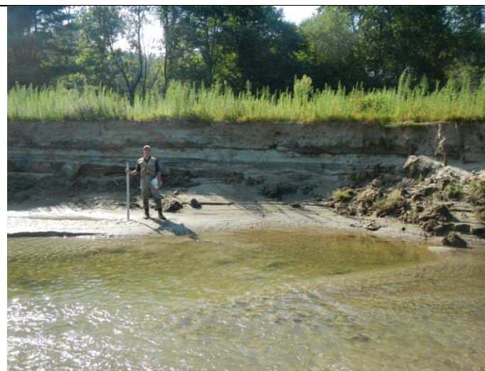
Eroding banks provide a large source of sediment
