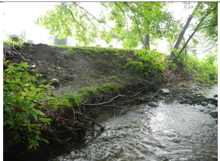
Bank scour along cemetery downstream from armor
