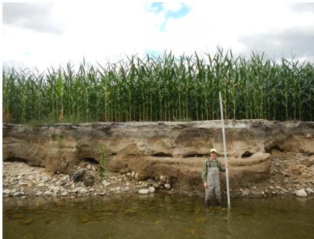
Figure 4.12: Major bank erosion in reach T5.01.
