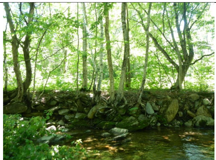
Historic bank armoring eliminated floodplain access
