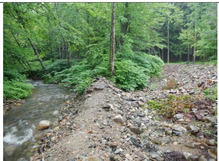
Berm cutting off access to flood chute by campground
