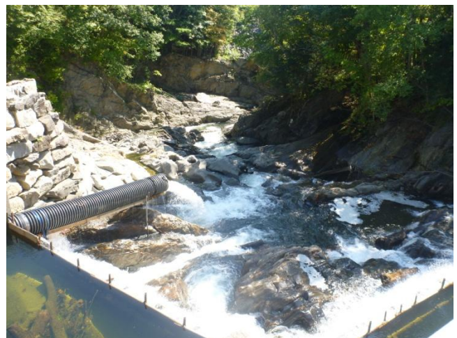
Figure 4.9: Brockway Mills Dam
