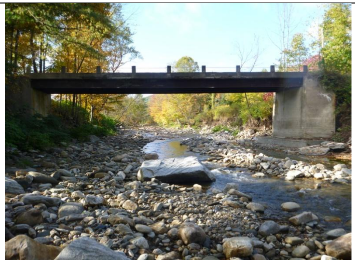
Channel working through July 2014 deposits
