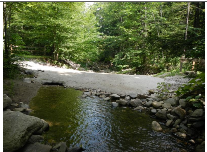
Channel aggrades enough to overtop old bridge
