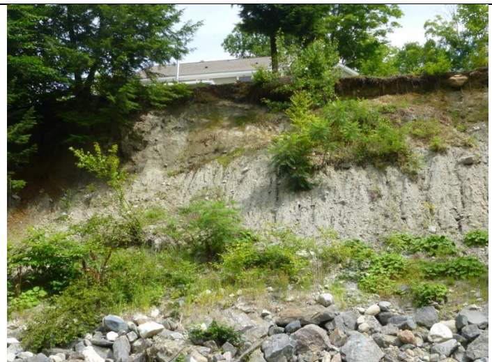
Mass failure posing future threat to home
