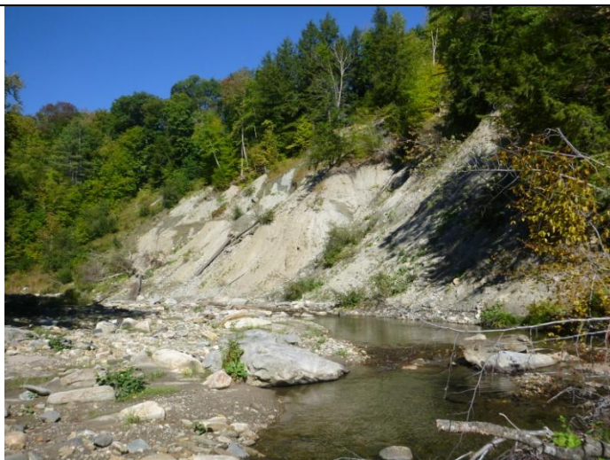
Multiple active mass failures present throughout T5.04
