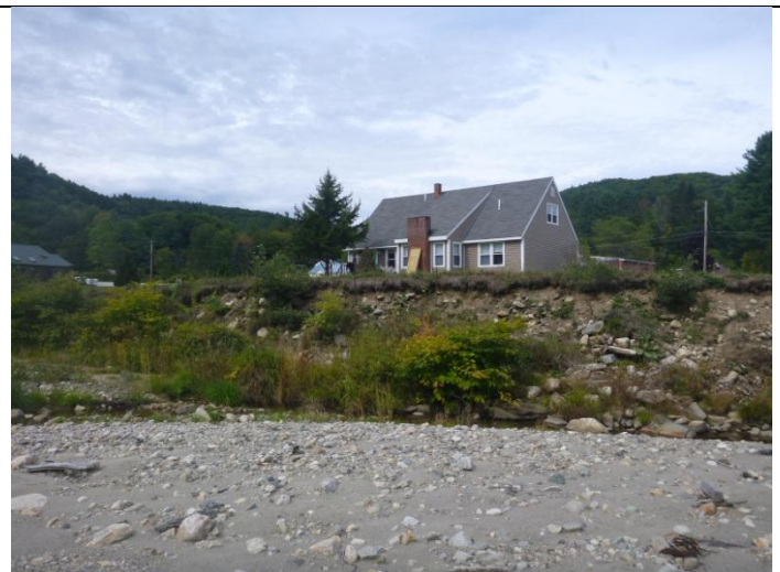
Banks are scoured and eroded from channel widening
