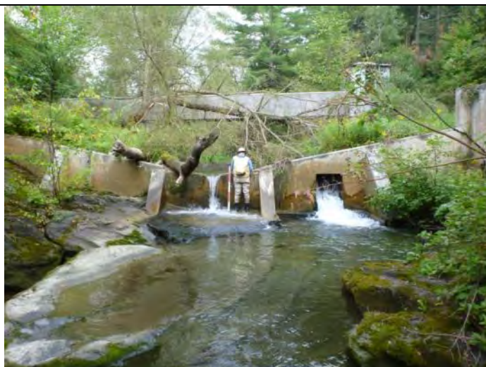
USGS weir and access bridge in lower reach
