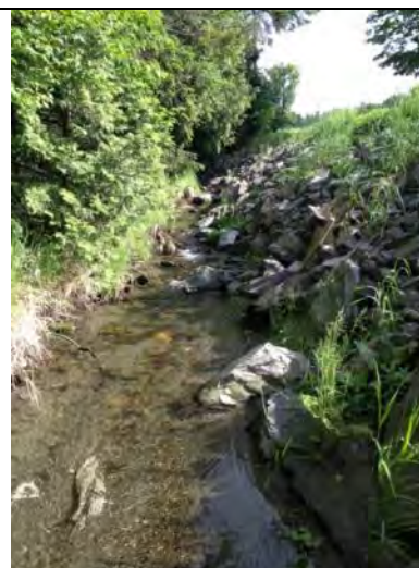
Armoring along Sheldon Brook Rd mid reach
