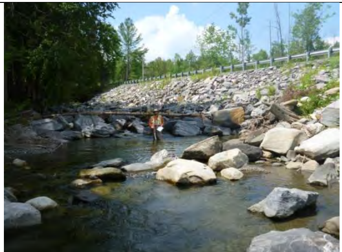
Large bed and bank armoring site in upper reach
