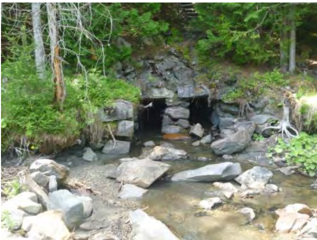
Figure 11: Extremely undersized stone culvert (left) leading to deep deposition of fine material and channel instability (right) on Whiteman Brook segment T3.7S1.06B.
