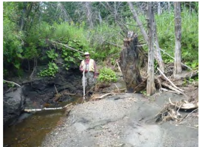
Figure 11: Extremely undersized stone culvert (left) leading to deep deposition of fine material and channel instability (right) on Whiteman Brook segment T3.7S1.06B.
