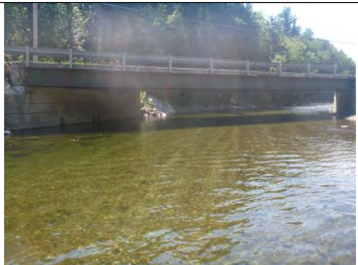
Goss Hollow Rd bridge - skewed and at a slope break, possible ice jam location
