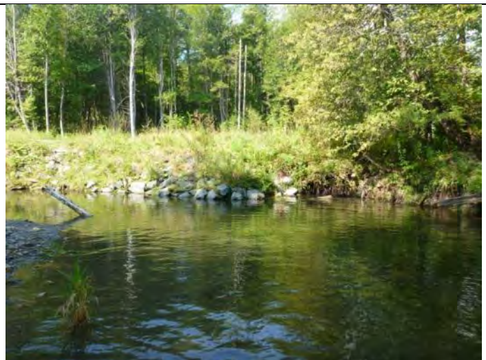
Failing armor along Water Andric Rd
