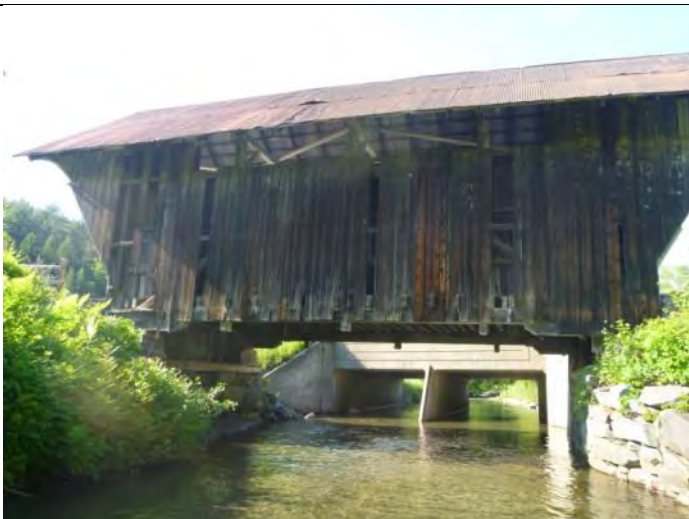
Schoolhouse covered bridge and South Wheelock Rd culvert in upper reach
