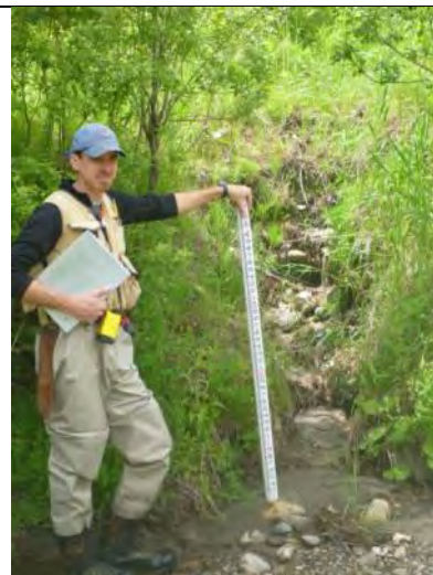
Small gully from a road ditch along New Boston Road
