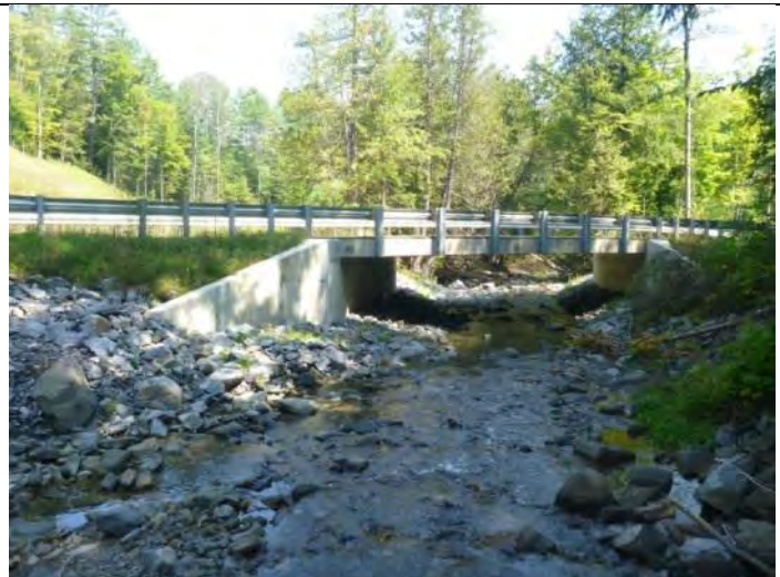
New Water Andric Rd bridge in lower segment
