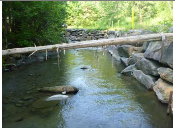
Stacked stone wall along Roy Rd
