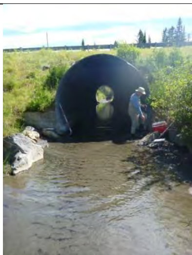
Culvert under Rt 2 near bottom of reach
