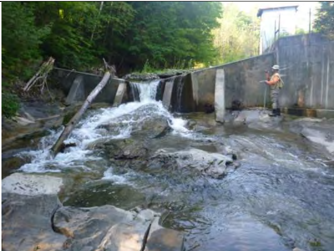
Abandoned USGS weir on a natural grade control
