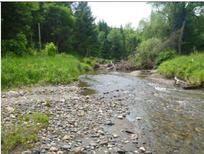
Failed cable bridge causing an unstable debris jam
