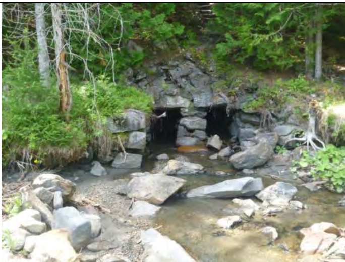
Stone culvert outlet
