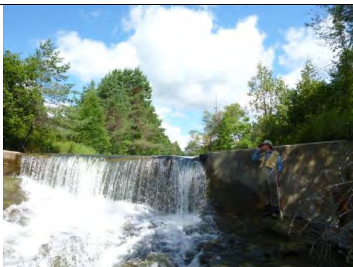
USGS weir over a bedrock grade control
