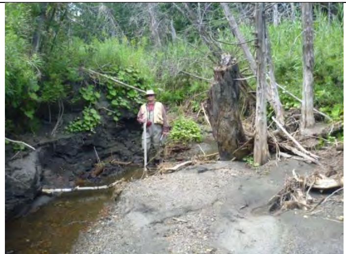
Deeply incised channel carving through sediments stored above culvert
