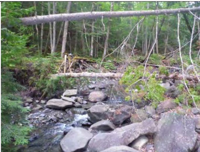
Channel degradation above the Trestle Rd culvert
