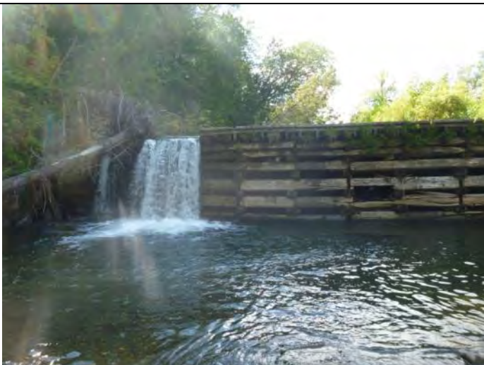
Timber crib dam at bottom of reach
