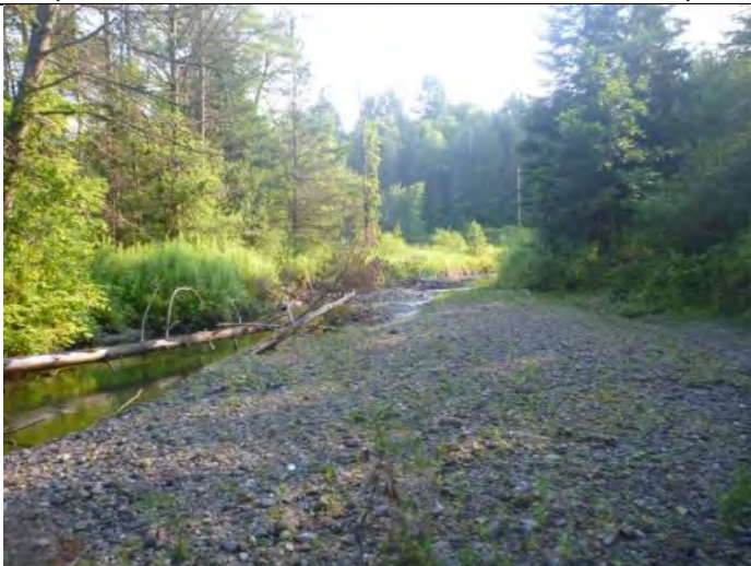
Gravel deposits below N Danville Rd culvert leading to Sleepers River T3.07
