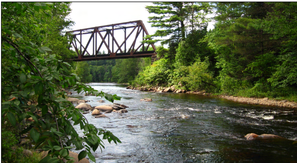
Figure 8: Railroad bridge, located in Reach M01.
