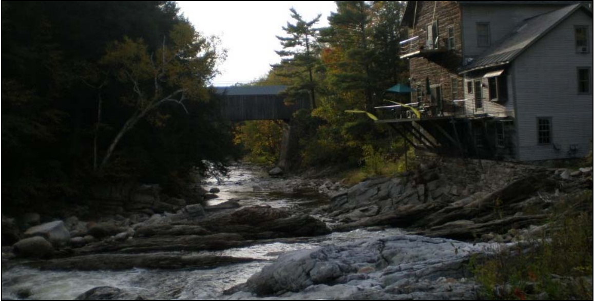
Figure 22. M03-B is a bedrock controlled segment at the site of the former Kingsley Mill.
