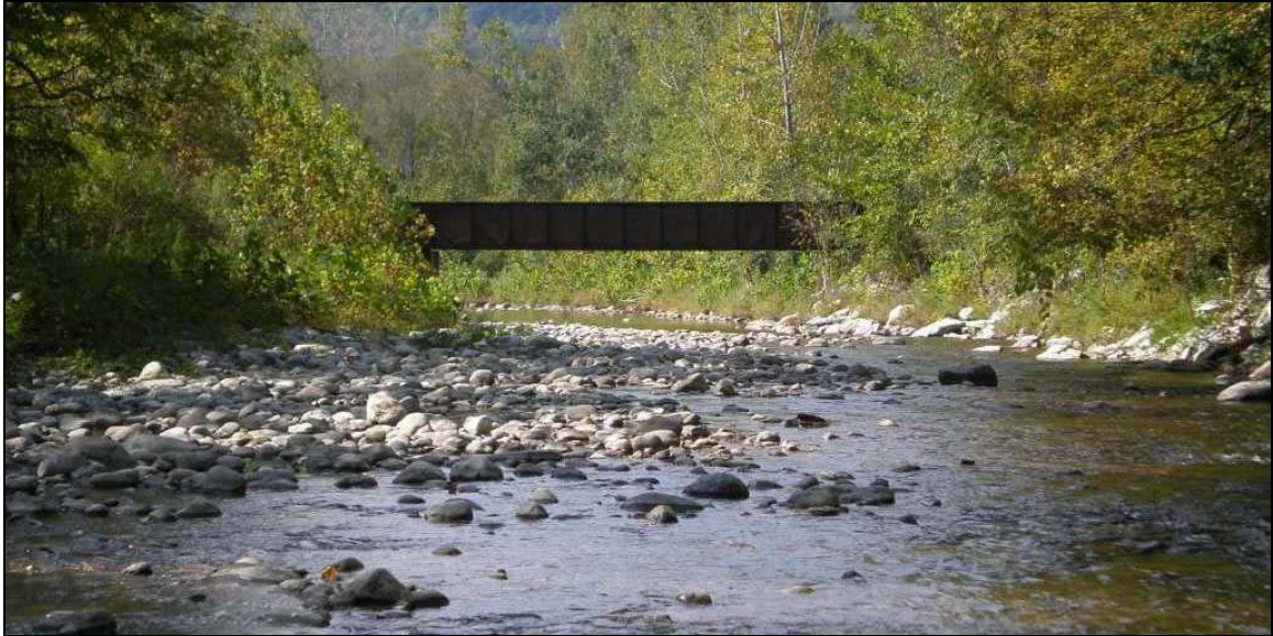
Figure 24. M01-B has been significantly impacted by channel straightening, berming, dredging, and armoring.
