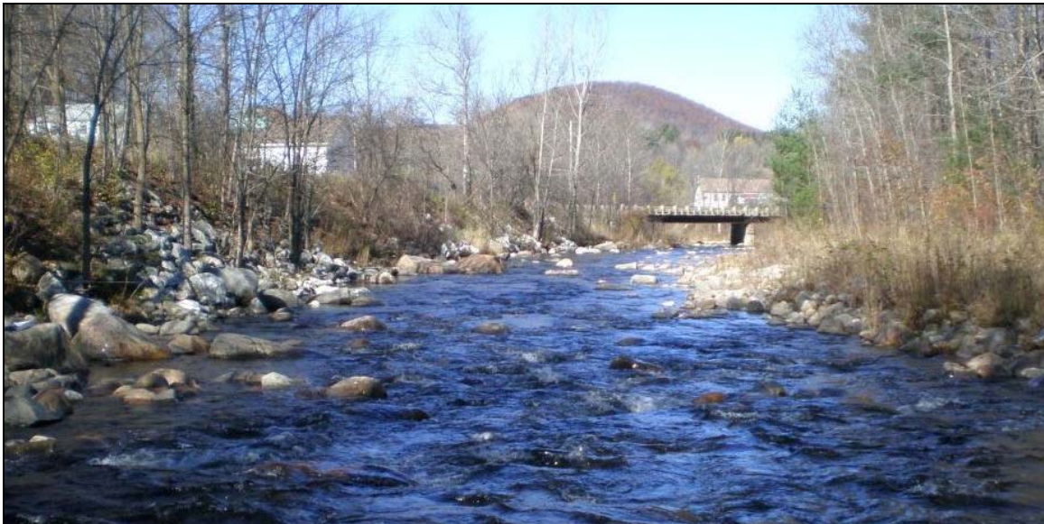
Figure 12. M10 has been historically straightened. There is a high degree of bank armoring within the reach.
