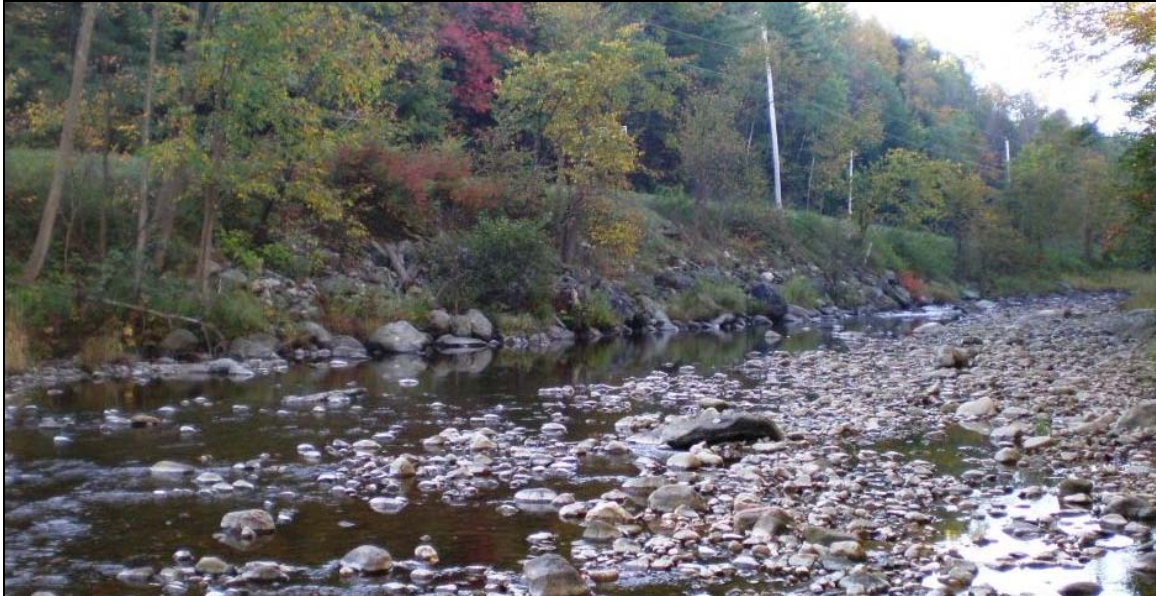
Figure 13. The valley width of M09 has been decreased due to encroachment from VT Route 103. The channel has undergone extreme widening.
