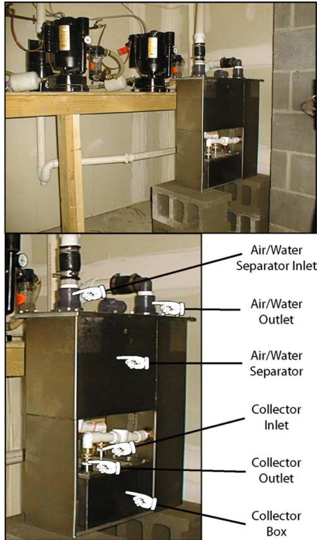
**Pilot Installations:** Two RME2000 amalgam separators were installed and observed in the pilot.
