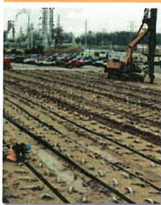
Above: Horizontal strip drains being placed after installation of wicks for a new maintenance facility on the Mississippi River floodplain in Memphis, TN.
