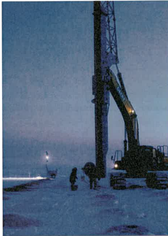
A total of 180,000 linear feet of wick drain was installed to 50 feet in sub-zero temperatures to accelerate drainage of soft compressible clay for the construction of an oil drilling platform in Prudhoe Bay, Alaska.
