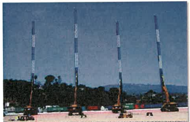
A total of 2,300,000 linear feet of wick drain was installed offshore (top photo) through as much as 40 feet of water, to depths up to 120 feet, and 8,800,000 linear feet of wick drain was installed on land (bottom photo), to depths of 98 feet, for the Port of Los Angeles Channel Deepening.
