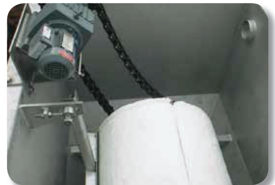
Internal view of an AquaDrum® cloth media filter
