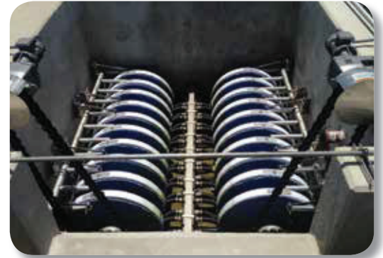
The modular design of the Aqua MiniDisk filter retrofits neatly into existing 9 ft. (2.74 m) wide concrete traveling bridge filter basins, providing more than two times the hydraulic capacity of the original sand filters.
