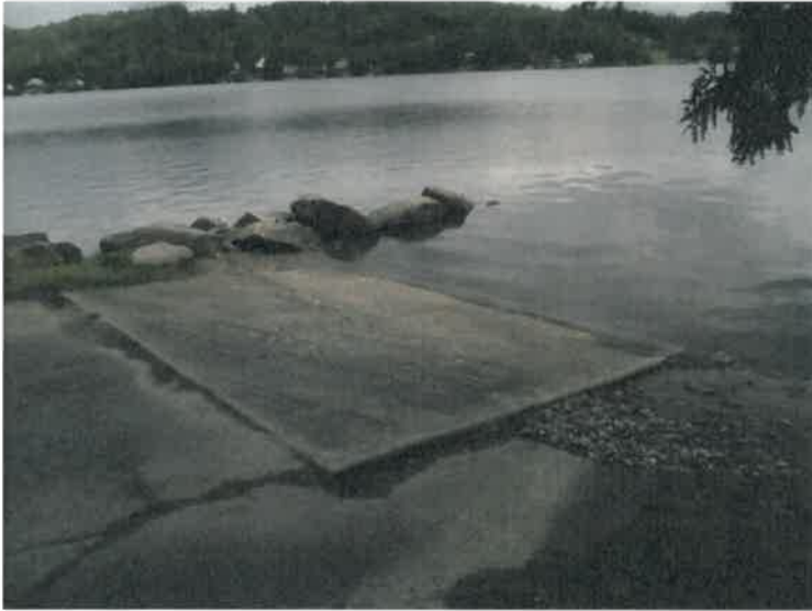
Photo 3: Ramp launch area facing north at stone breakwater.
