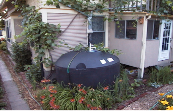
Above Ground Cistern
