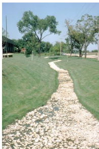
Infiltration Trench
