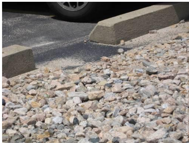
A gravel diaphragm catches runoff and distributes it as sheet flow to the filter strip, settling out sediment and preventing erosion.
