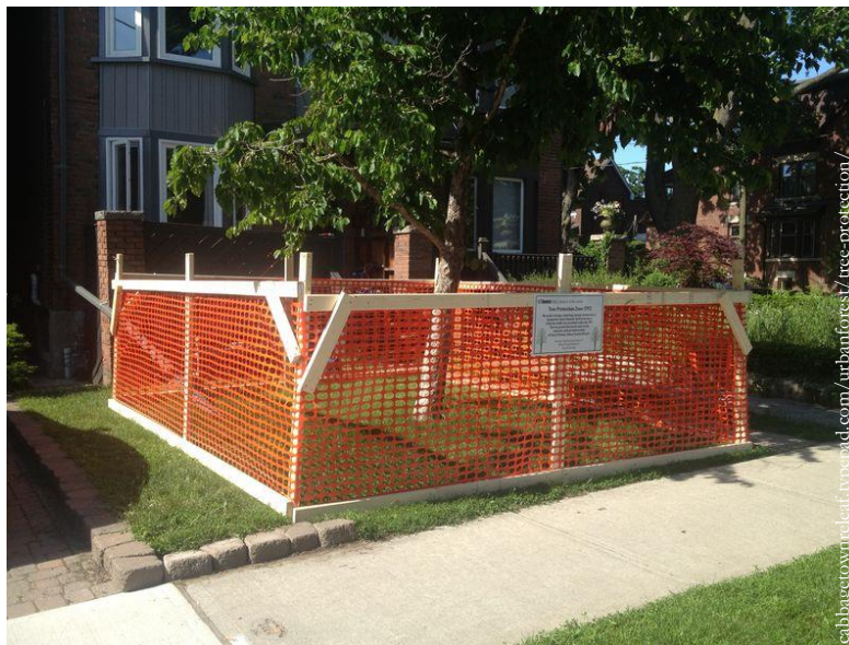
Protecting trees to be retained from damage and disturbance during construction activities is critically important for the trees' long-term health and performance.
