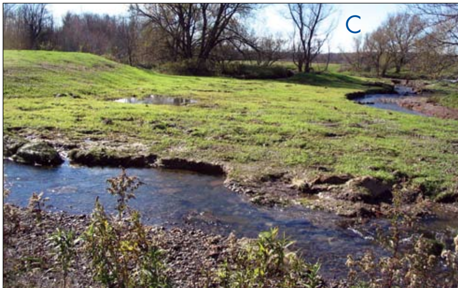
Figure 15. Flood plain restoration project on Rugg Brook in the St. Albans Bay watershed. (A) Rugg Brook before restoration showing incised and eroding stream channel. (B) Construction in progress. (C) Rugg Brook with restored access to its flood plain after completion of the project. Source: Vermont Department of Environmental Conservation River Management Program.
