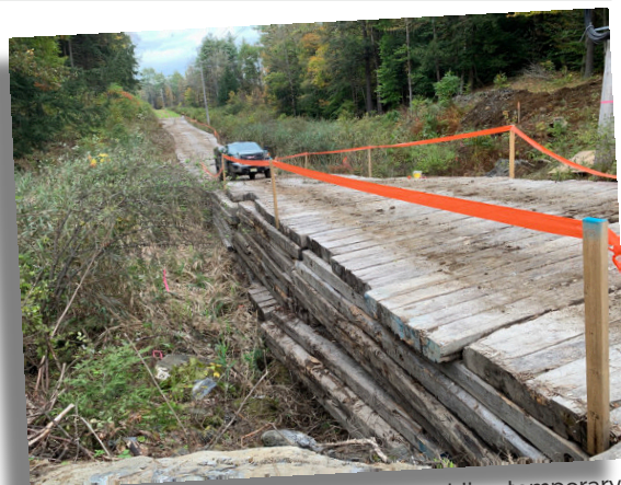
Layered wetland matting providing temporary wetland crossing
