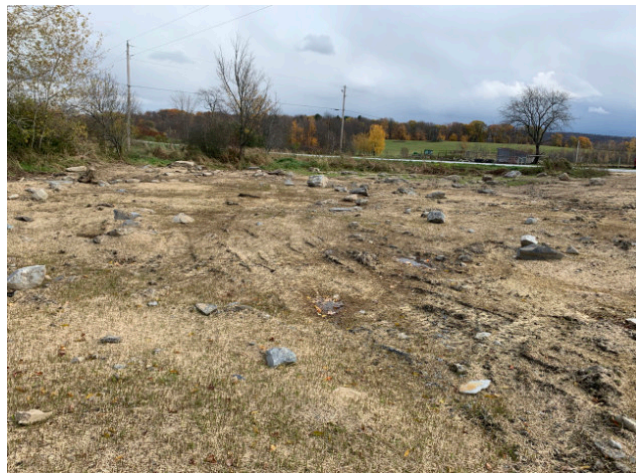
Post restoration-fill removed, rough finish incorporating boulders
