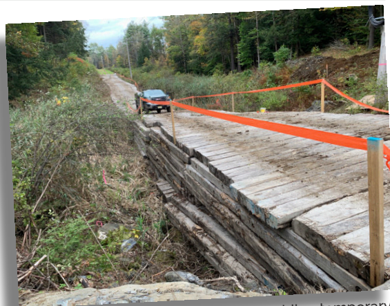
Layered wetland matting providing temporary wetland crossing
