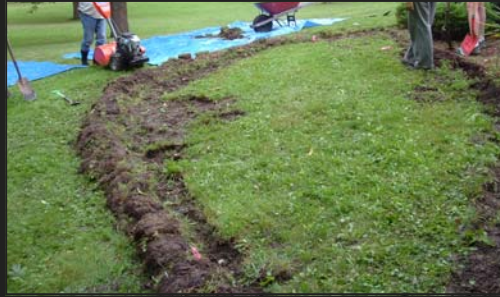
Build the berm with sod
