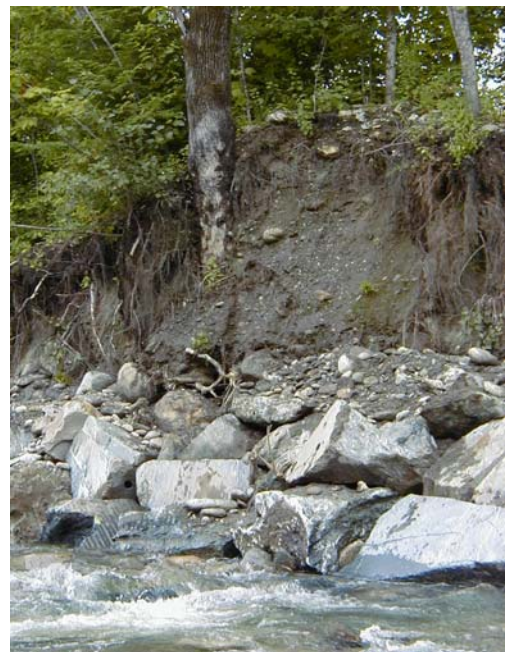
Figure 6.8C Example of berm and streambank armoring with stone wall. Dirt on top of stone wall is an old berm; note large tree growing in berm that was present before berm was constructed. Saplings on top of berm have grown up since berm was built several decades ago. Berm height above average water level is approximately 10 feet.
