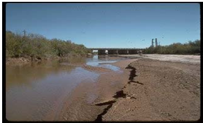
Figure 6.3B Poor pool substrate condition
