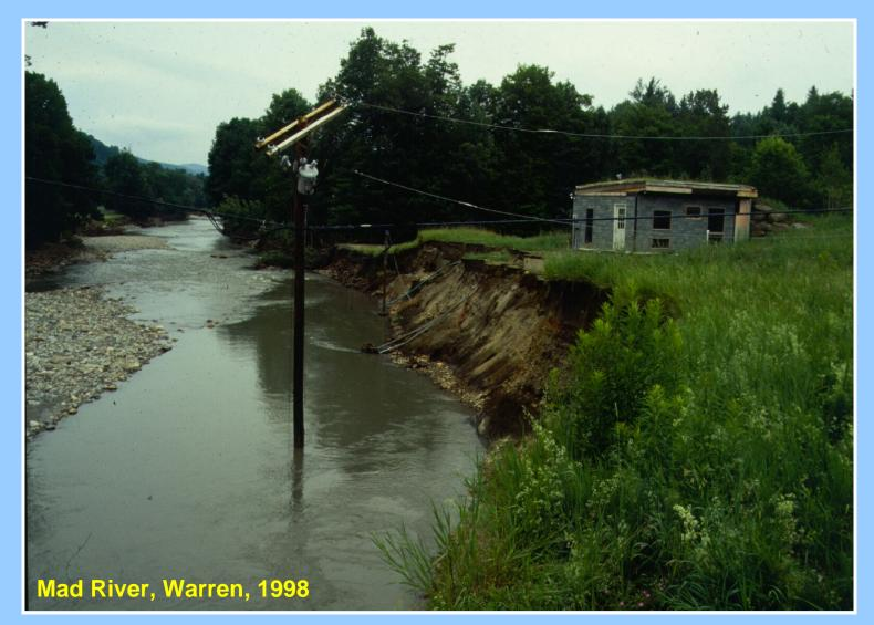
Home built 100 ft from NFIP Floodway and 8 ft Above Q100; Channel Adjustment Occurred Overnight
