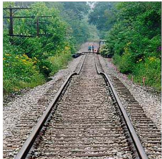
Longwall subsidence from coal mining undermines this railway in western Pennsylvania. Image credit: Pennsylvania Department of Environmental Protection.
