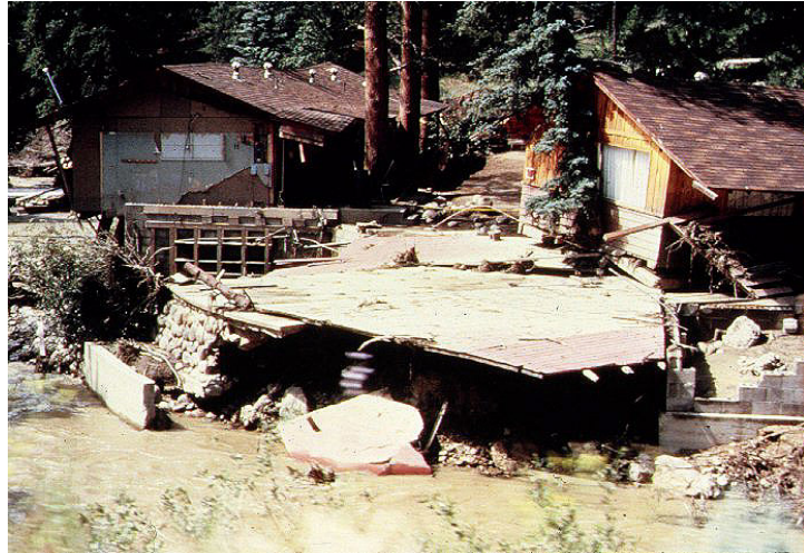
Campground lodge buildings following failure of the Lawn Lake Dam, Rocky Mtn. Nat'l. Park. Image credit: Estes Park, Colorado.
