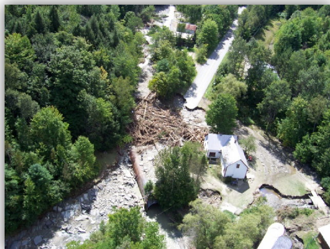
Figure 6: Tree dam that formed during the flood Source: VTRANS
