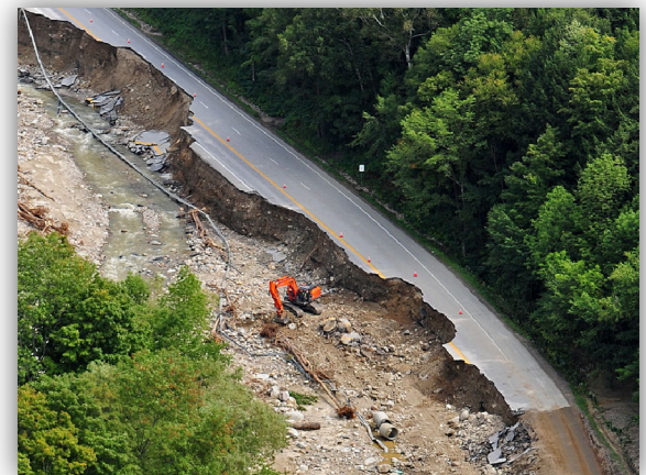
Figure 1: VT Route 107 Source: VTRANS
