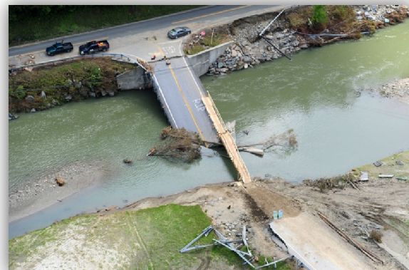
Figure 2: Rochester pedestrian foot bridge
