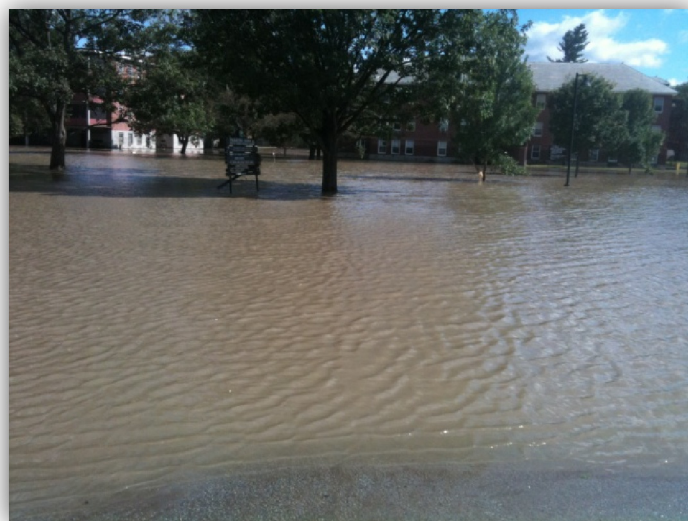
Figure 3: State Office Complex Flooding, Waterbury Source: VT ANR
