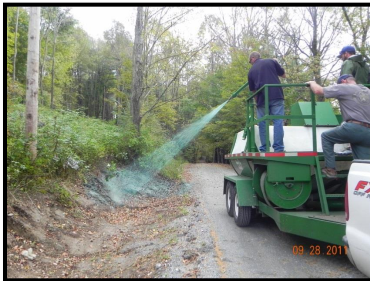
The Town of Pawlet road crew using the hydroseeder to seed newly ditched roadway in Pawlet.
