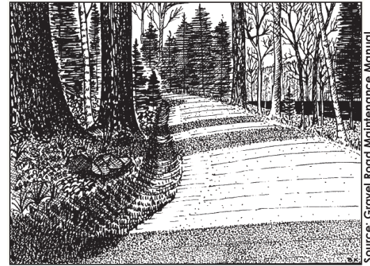
Crowned driveway with a rock-lined drainage ditch.
