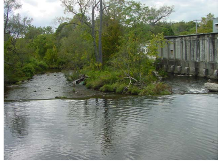
Bridge Name: Paper Mill Bridge (covered) Photo No.: DSC00061.JPG Date: 9/21/2006 View/Description: D/S, View of river below bridge
