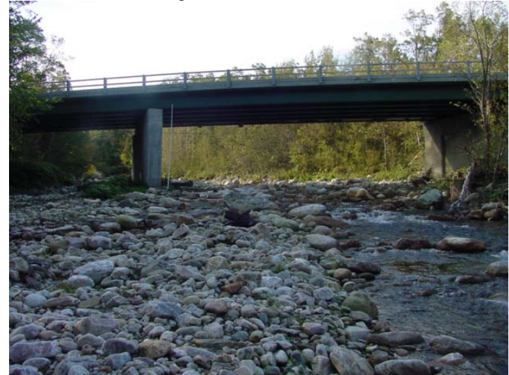
Bridge Name: Route 9, Bennington Photo No.: DSC00091.JPG Date: 9/22/2006 View/Description: U/S, View of outlet
