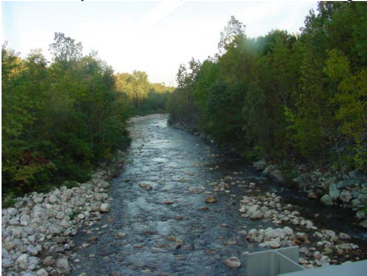
Bridge Name: Park Street Photo No.: DSC00079.JPG Date: 9/22/2006 View/Description: D/S, View of main channel at bridge
