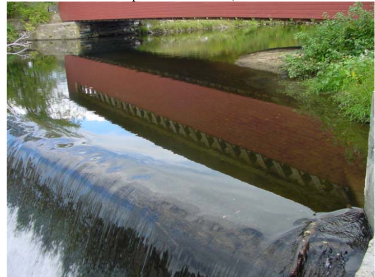
Bridge Name: Paper Mill Bridge (covered) Photo No.: DSC00062.JPG Date: 9/21/2006 View/Description: U/S, View of outlet
