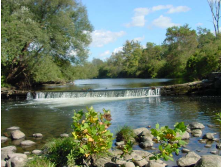
Bridge Name: Henry Bridge Photo No.: DSC00054.JPG Date: 9/21/2006 View/Description: U/S, View of river above bridge
