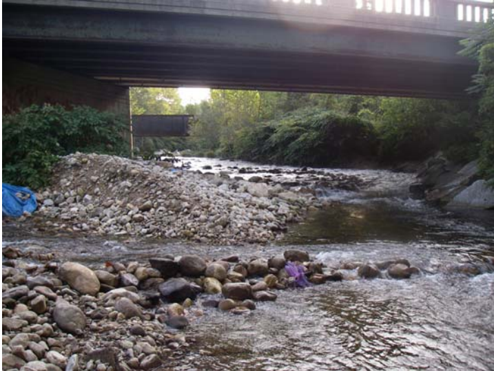
View/Description: U/S, View of left cell of bridge
