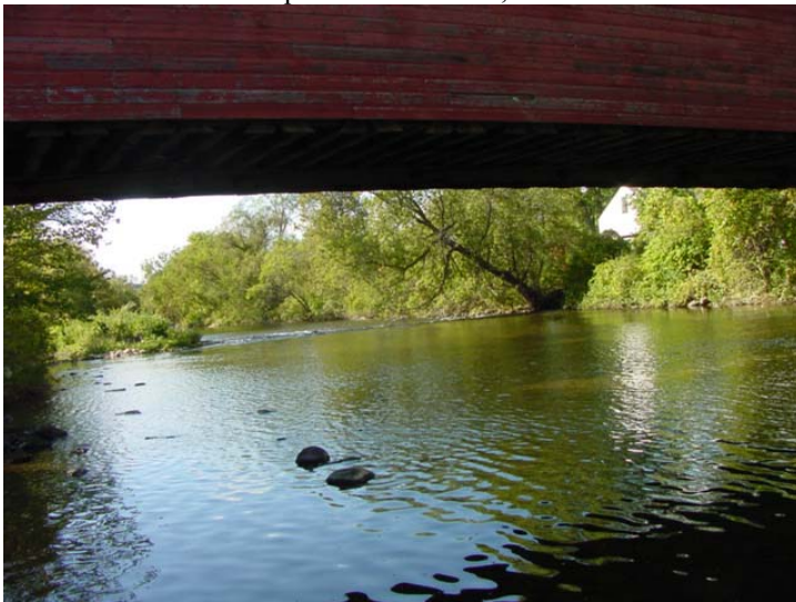
Bridge Name: Henry Bridge Photo No.: DSC00056.JPG Date: 9/21/2006 View/Description: D/S, View of inlet
