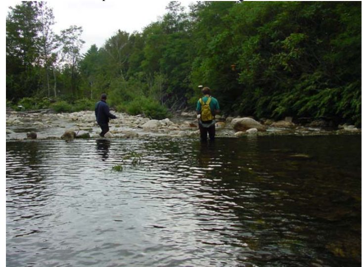
Reach/Segment: M06T3.03 Photo No.: DSC00030.JPG Date: 9/6/2006 View/Description: Man-made grade control D/S
