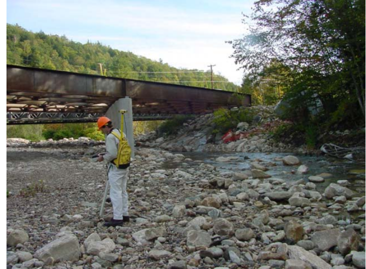
Bridge Name: Route 9, Woodford Photo No.: DSC00096.JPG Date: 9/22/2006 View/Description: U/S, View of outlet
