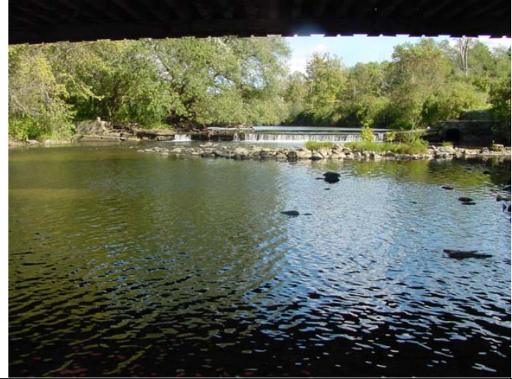
Bridge Name: Henry Bridge Photo No.: DSC00057.JPG Date: 9/21/2006 View/Description: U/S, View of outlet
