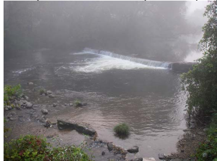
Reach/Segment: M02 Photo No.: 32-2426 Date: 9/20/2006 View/Description: U/S View of weir upstream of Henry Bridge
