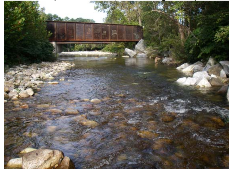
Bridge Name: Railroad Bridge Photo No.: IMG2462.JPG Date: 9/22/2006 View/Description: D/S, View of bridge from upstream
