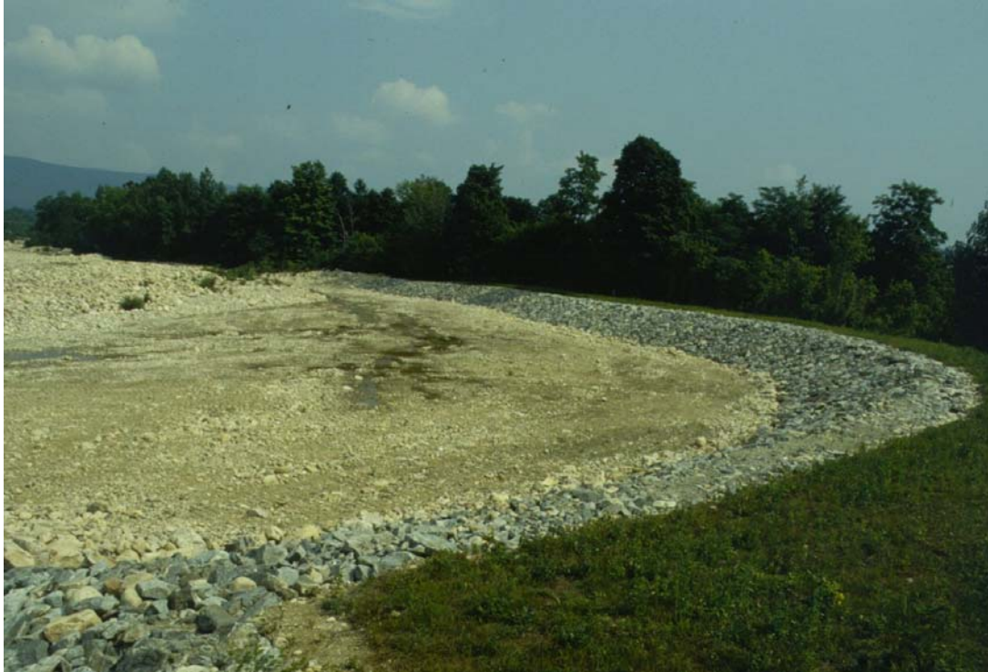
Plate 5: Bank Armoring Following 1987 Flood, Roaring Branch Upstream of Park St. Bridge.
