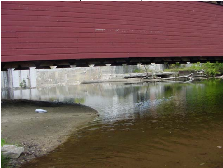
Bridge Name: Paper Mill Bridge (covered) Photo No.: DSC00060.JPG Date: 9/21/2006 View/Description: D/S, View of inlet
