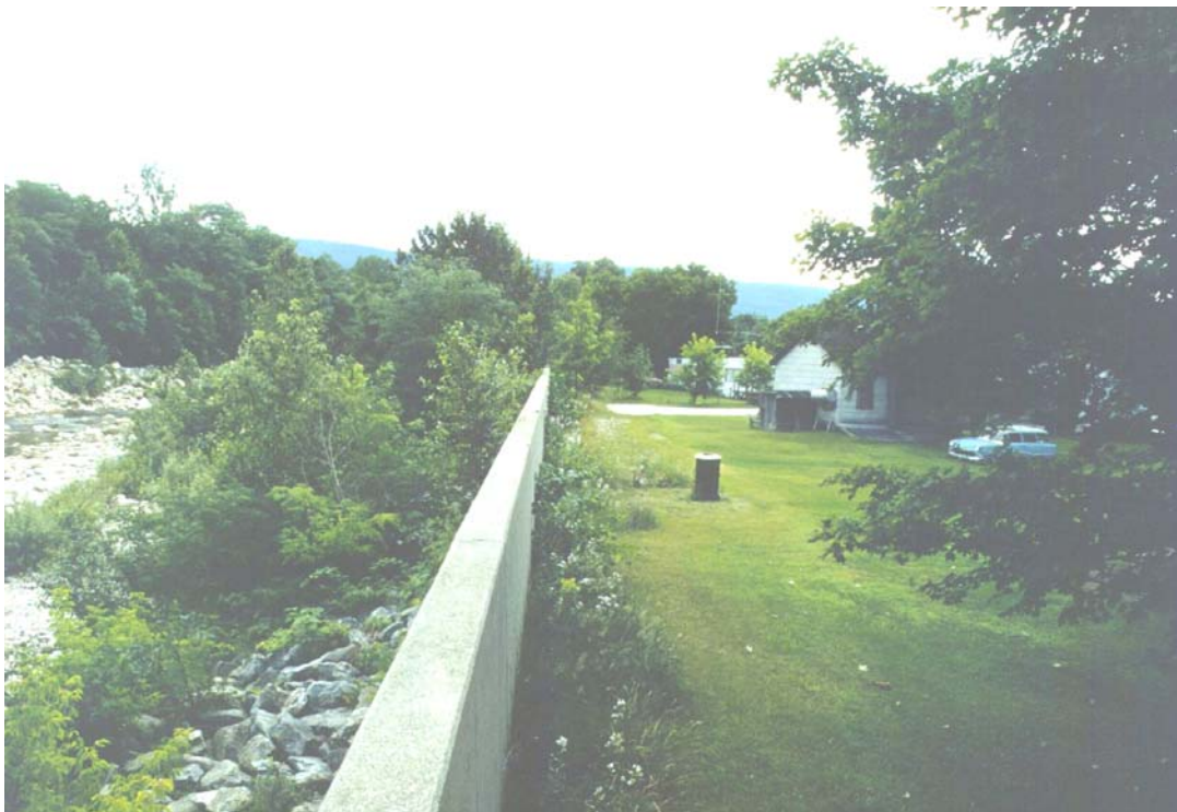
Plate 2: USAOCE Floodwall Downstream of Brooklyn Bridge.
