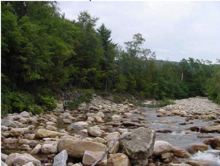
Reach/Segment: M06T3.03 Photo No.: DSC00036.JPG Date: 9/6/2006 View/Description: RB Erosion
