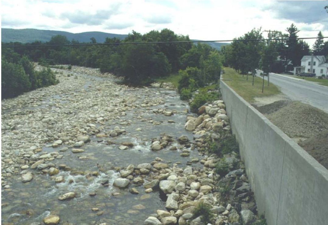
Plate 1: USACOE Floodwall Upstream of Brooklyn Bridge, 1987
