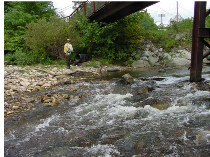
Reach/Segment: M06b Photo No.: DSC00031.JPG Date: 9/20/2006 View/Description: D/S culvert
