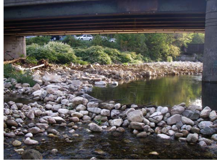
View/Description: U/S, View of center cell of bridge
