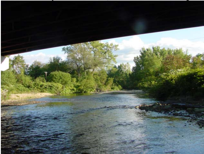
Bridge Name: State Route 279 Photo No.: DSC00074.JPG Date: 9/21/2006 View/Description: U/S, View of river above bridge
