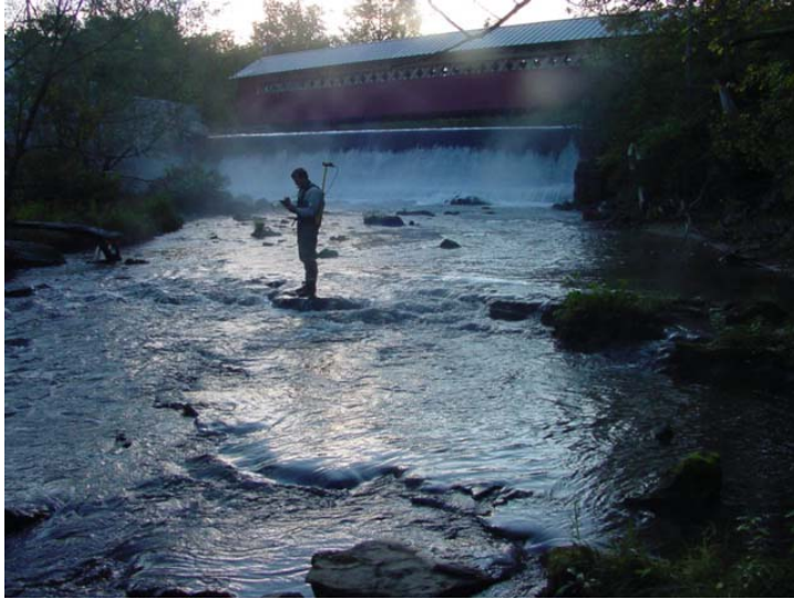
Reach/Segment: M03 Photo No.: DSC00049.JPG Date: 9/21/2006 View/Description: U/S Paper Mill Dam (bedrock)
