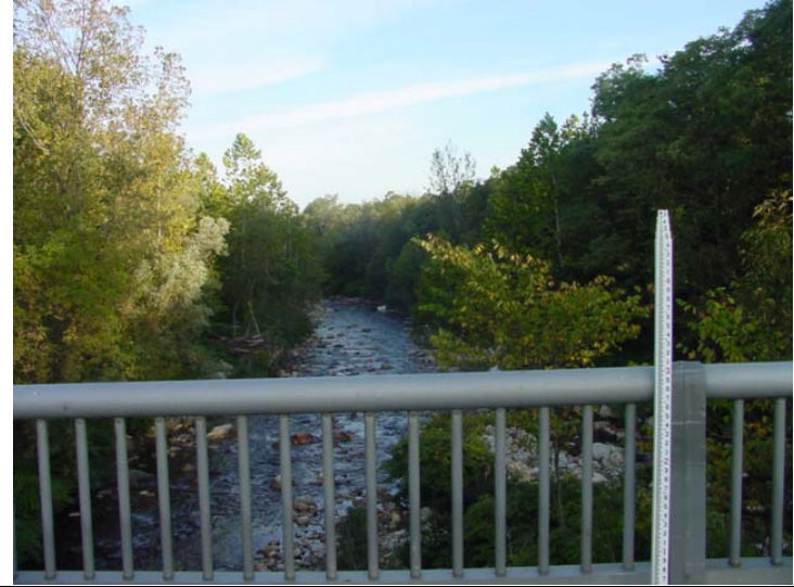
Bridge Name: Brooklyn Bridge Photo No.: DSC00086.JPG Date: 9/22/2006 View/Description: D/S, View of channel
