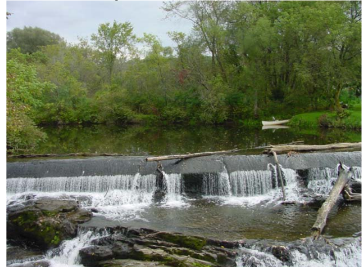
Reach/Segment: M04 Photo No.: DSC00044.JPG Date: 9/20/2006 View/Description: U/S Reach break at weir
