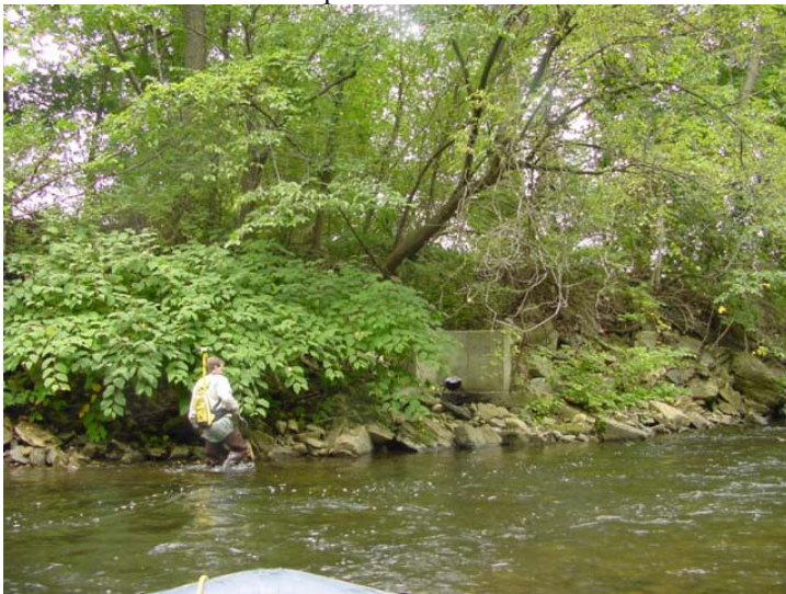
Reach/Segment: M06b Photo No.: DSC00029.JPG Date: 9/20/2006 View/Description: RB culvert
