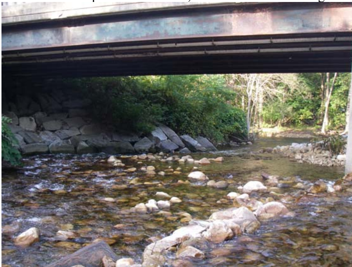
Bridge Name: Benmont Avenue Photo No.: IMG2457.JPG Date: 9/22/2006 View/Description: D/S, View of left cell of bridge
