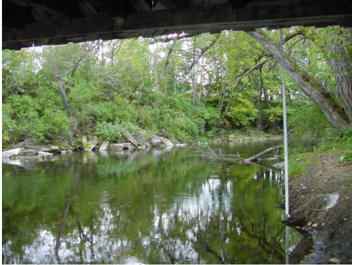
Bridge Name: Silk Road Bridge (covered) Photo No.: DSC00067.JPG Date: 9/21/2006 View/Description: D/S, View of river below bridge
