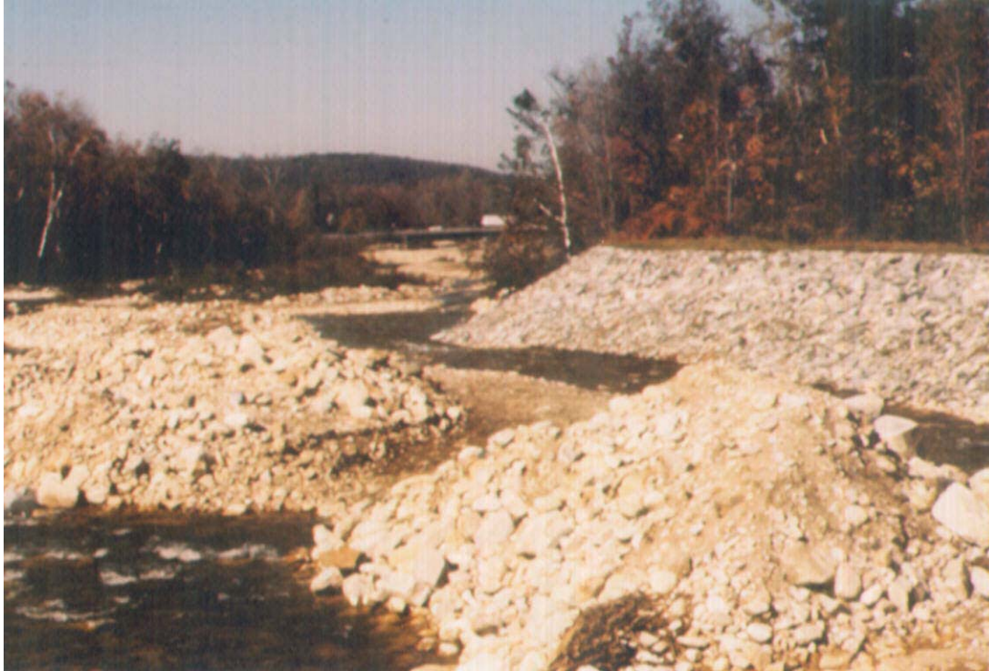
Plate 15: Roaring Branch, behind Veterans Home Looking Upstream, 1988.
