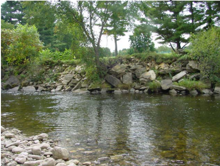
Reach/Segment: M06b Photo No.: DSC00033.JPG Date: 9/20/2006 View/Description: LB revetment near golf course
