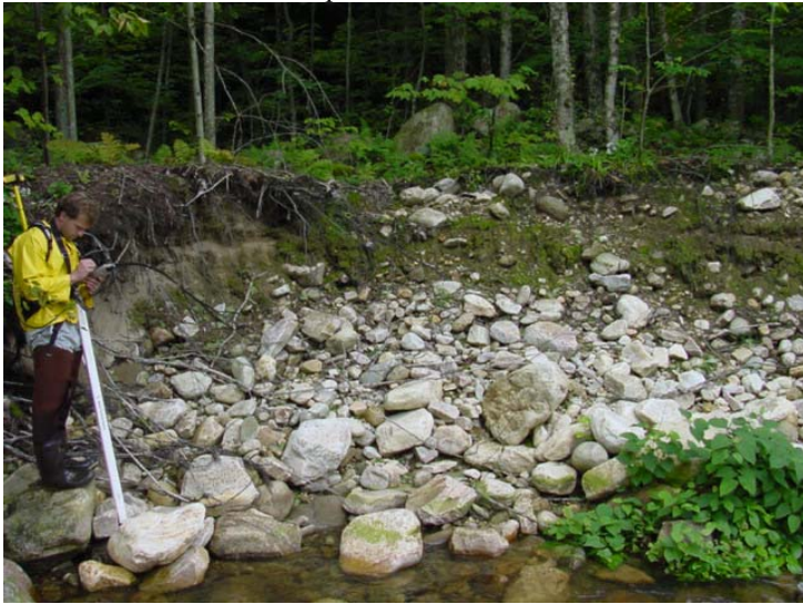
Reach/Segment: M06T3.04 Photo No.: DSC00011.JPG Date: 9/5/2006 View/Description: LB Erosion
