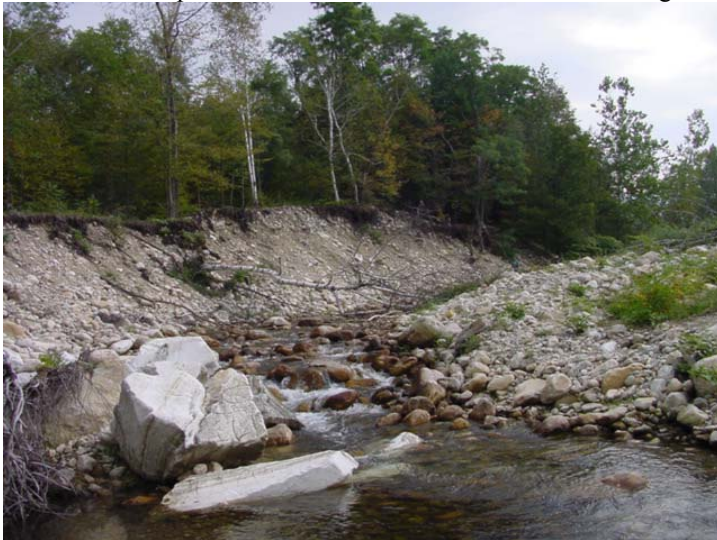
Reach/Segment: M06T3.01 Photo No.: DSC00010.JPG Date: 9/19/2006 View/Description: U/S Erosion near Park St. Bridge
