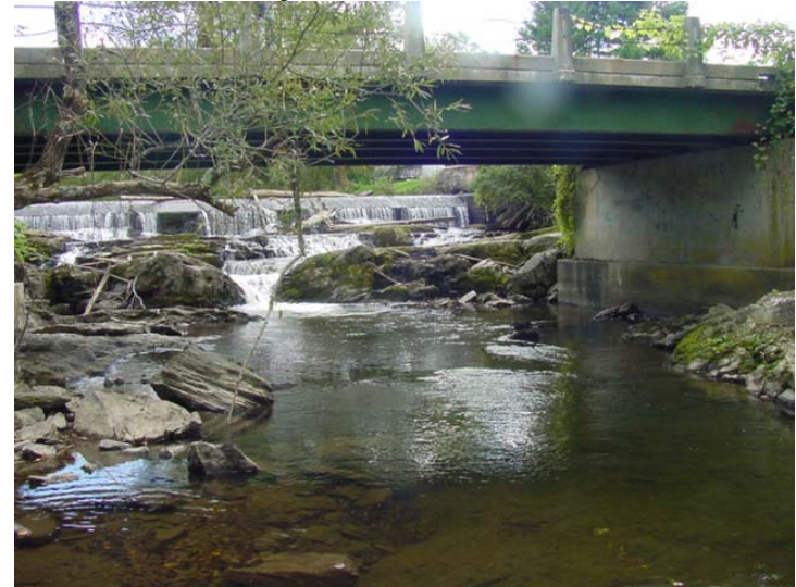
Bridge Name: Murphy Road Bridge (west) Photo No.: DSC00066.JPG Date: 9/21/2006 View/Description: U/S, View of outlet
