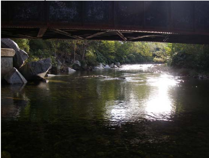
Bridge Name: Railroad Bridge Photo No.: IMG2460.JPG Date: 9/22/2006 View/Description: U/S, View of outlet from downstream
