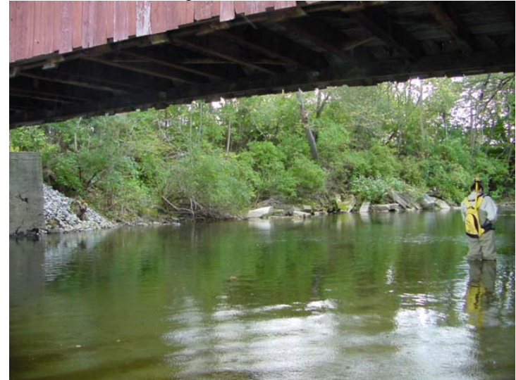
Bridge Name: Silk Road Bridge (covered) Photo No.: DSC00070.JPG Date: 9/21/2006 View/Description: D/S, View of inlet
