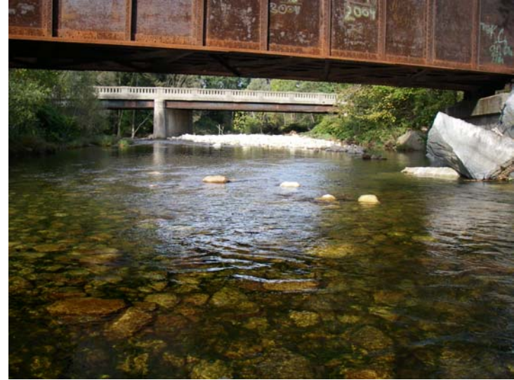
Bridge Name: Railroad Bridge Photo No.: IMG24561.JPG Date: 9/22/2006 View/Description: D/S, View of inlet from upstream
