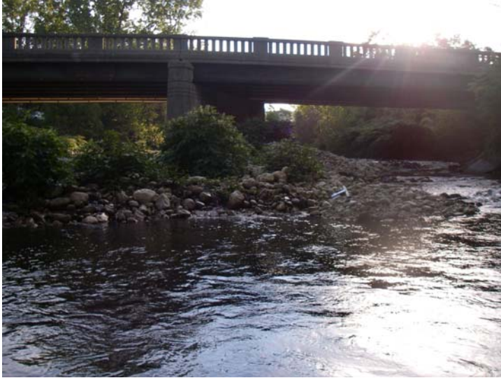
View/Description: U/S, View of bridge from downstream
