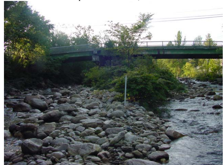
Bridge Name: Brooklyn Bridge Photo No.: DSC00087.JPG Date: 9/22/2006 View/Description: U/S, View of outlet
