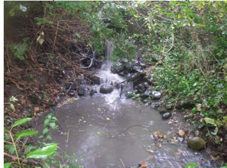
Reach/Segment: M03 Photo No.: 31-2425 Date: 9/20/2006 View/Description: U/S Outfall under Bennington Road
