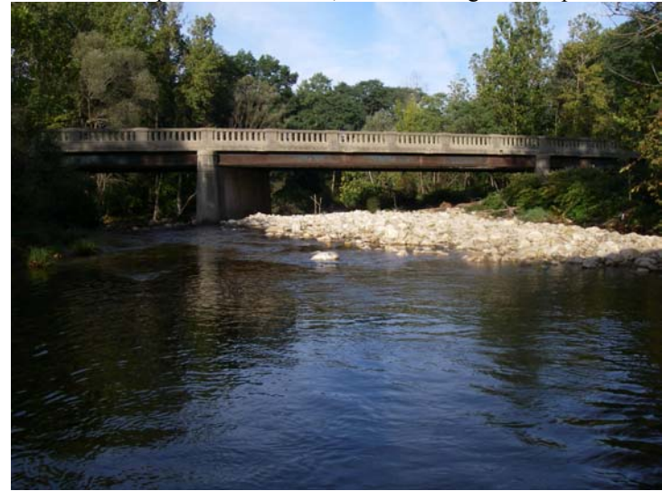
Bridge Name: Benmont Avenue Photo No.: IMG2458.JPG Date: 9/22/2006 View/Description: D/S, View of bridge from upstream
