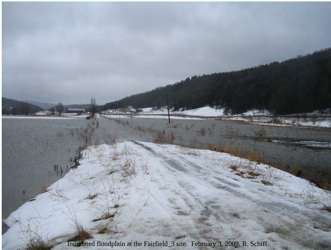
FIGURE 2 Floodplain Inundation along Black Creek
