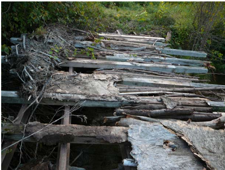
Figure 3. LaRue private bridge, Reach M17, Segment B 10 September 2007
