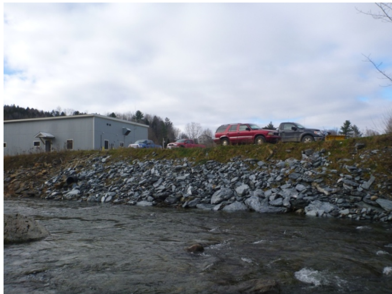
Figure 25: Left bank armoring and development
