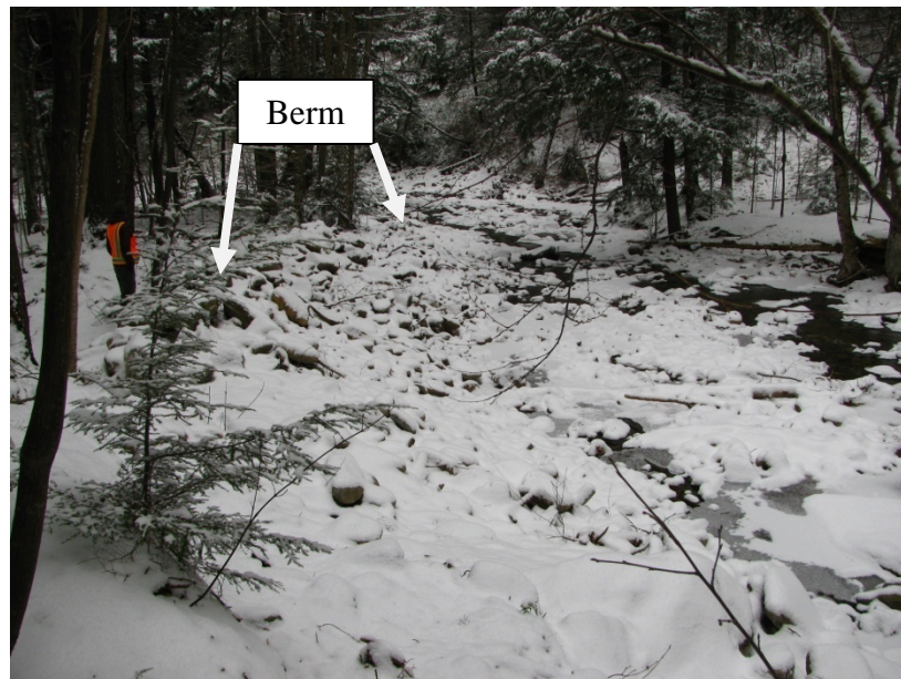
Figure 6: Berming along the left bank in Reach M12
