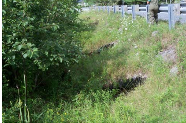
Figure 4.76. Three culverts at Route 244 Crossing
