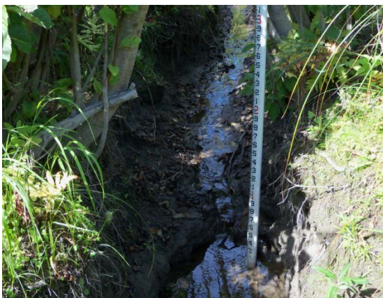
Figure 4.56 Active head cut in clay soils in swale
