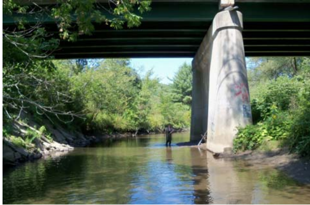
Figure 4.75. Center pier of Route 244 Bridge
