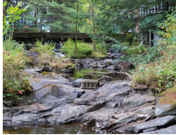
Figure 4.29 Looking upstream at natural ledge & Dam
