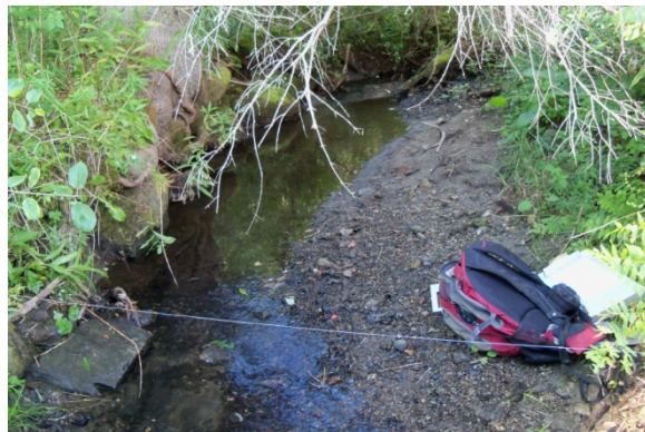
Figure 4.47 Channel straightening and bank armoring
