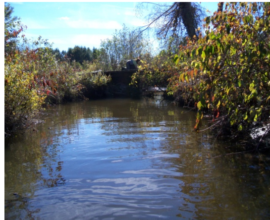
Figure 4.52 Impounded channel below farm bridge
