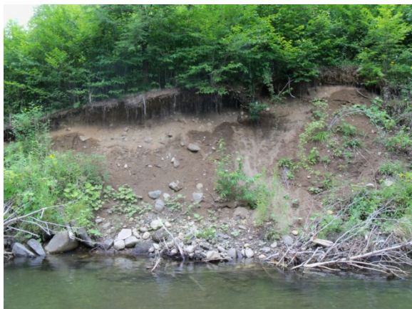
Figure 4.19 Mass failure on east bank
