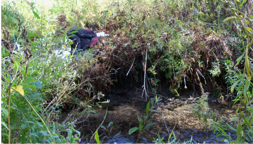
Figure 4.39 Bank erosion indicative of channel widening in segment R16T2.05-D
