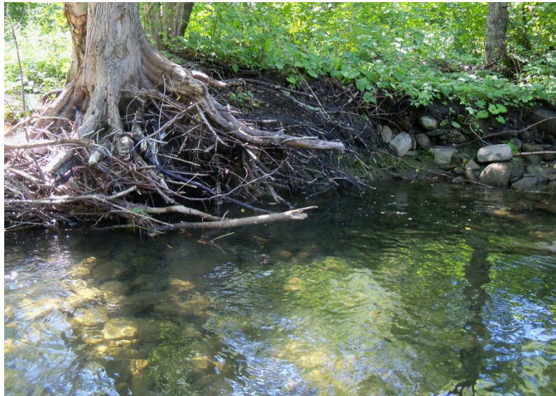
Figure 4.66 Tree root is providing a stable undercut bank
