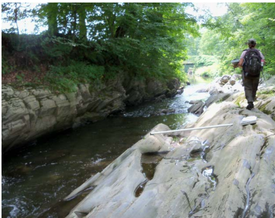
Figure 4.14 Ledge grade control above Geer dam
