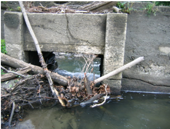
Figure 4.3 Constriction at dam in R15-B (Looking downstream)
