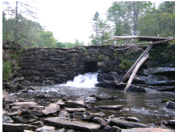
Figure 4.4 Constriction at dam in R15-B (looking upstream)
