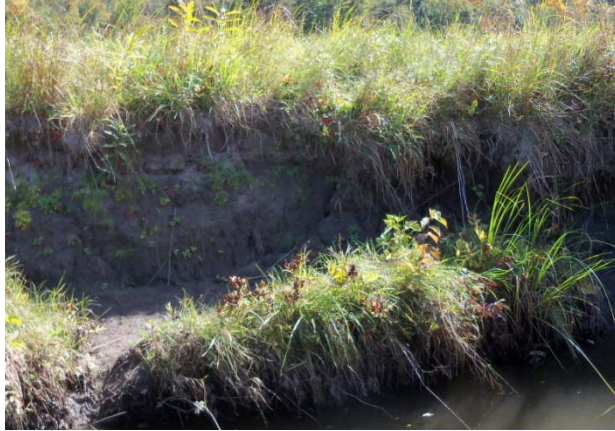
Figure 4.58 Bank erosion and lack of buffer
