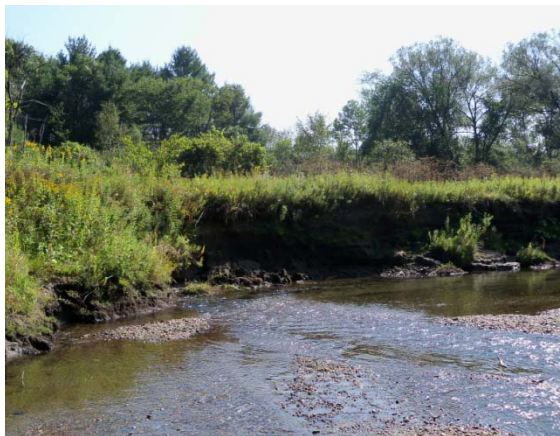
Figure 4.8 Extensive bank erosion in Reach R17
