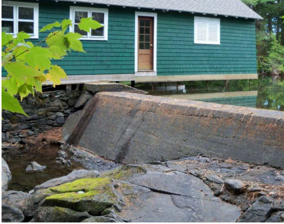
Figure 4.28 Lake Fairlee Dam from downstream
