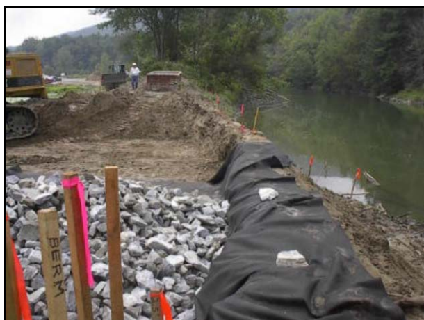
Northern end of berm at the site of former lagoon area, looking south. Left: lowering of the berm and placement of rip-rap for drainage during remediation in 2004 (from Metcalf & Eddy, 2005). Right: revegetation observed during Phase 2 assessment.
