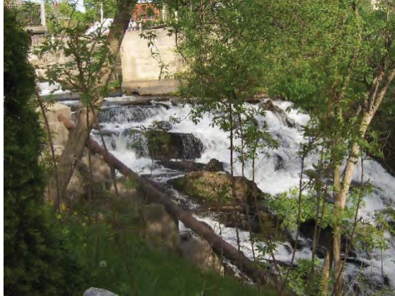
Figure 7.2. Dam and waterfall in downtown Brandon on Reach M02 (BCE, 5/7/2010)
