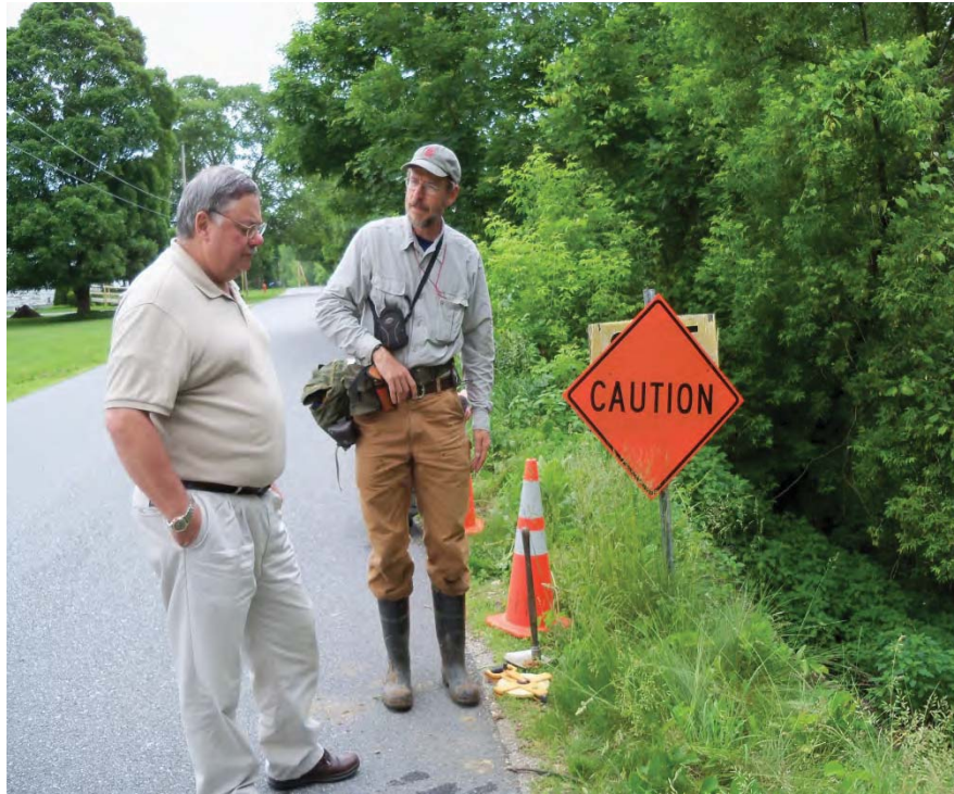
Figure 7.22. George Springston (Vermont Geological Survey) and Keith Arlund (Brandon Town Manger) examine the mass failure on Wheeler Rd (BCE, 5/25/2011)
