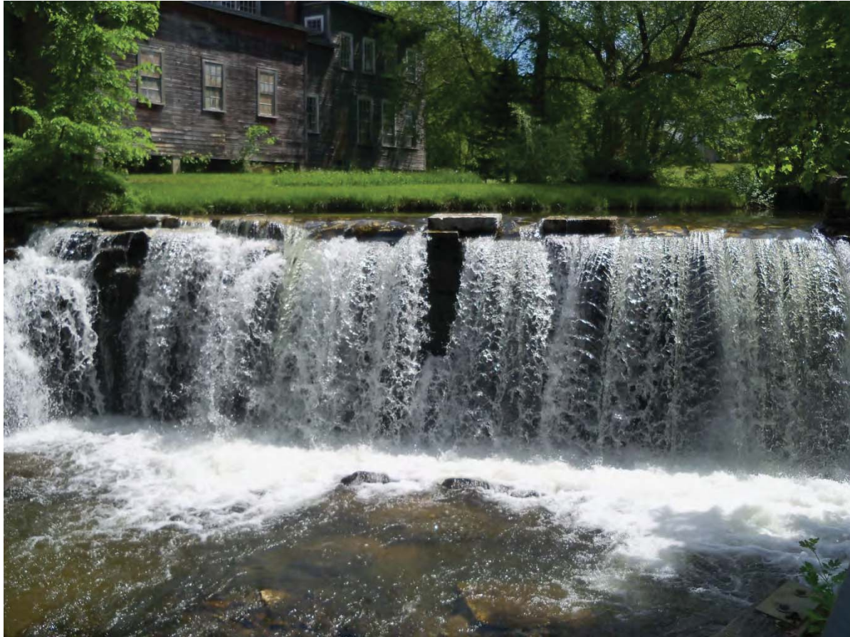
Figure 7.21. Dam on Neshobe River in downtown Brandon (BCE, 5/25/2011)
