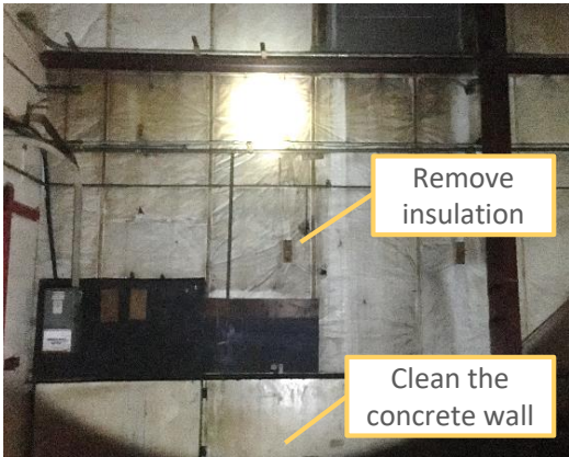
Photo 1: Concrete wall and insulation
