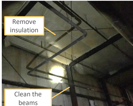
Photo 2: Insulation on wall and ceiling
