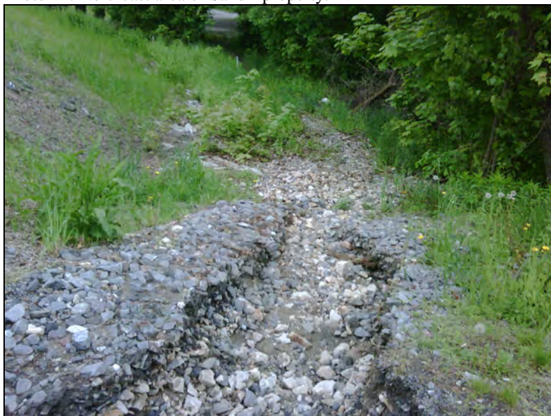
Photo #3: Looking east down trail/property line.
