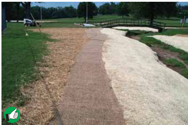
Excellent soil coverage at stabilization project using hand scattered straw, jute matting, and erosion blanket.
