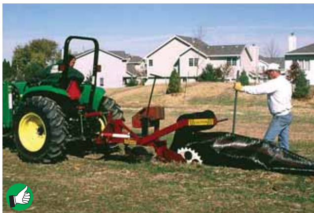
Tractor mounted silt fence slicing devices cut a slit into the ground and push fabric in. Installation is quicker and performance is better than the open trench method, making this approach attractive for large sites.
