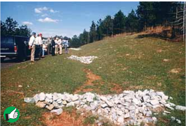
Good installation of temporary rock silt checks. Remember to tie sides of silt check to upper banks. Middle section should be lower. Clean out sediment as it accumulates. Remove silt checks after site and channel are stabilized with vegetation.
