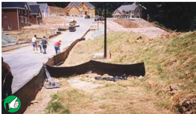
Excellent example of J-hook installation to intercept muddy runoff flowing along silt fence. Good temporary seeding and mulching (right side).
