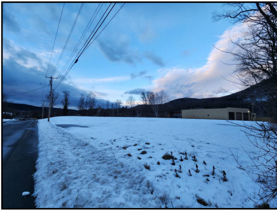
9: View of the Former Robertson Paper Mill, facing north.
