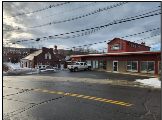
12: View of adjoining commercial buildings from Bridge Street, facing northwest.
