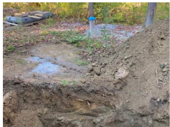
Photo #6 : View of TP-3, located south of the well, facing north.
