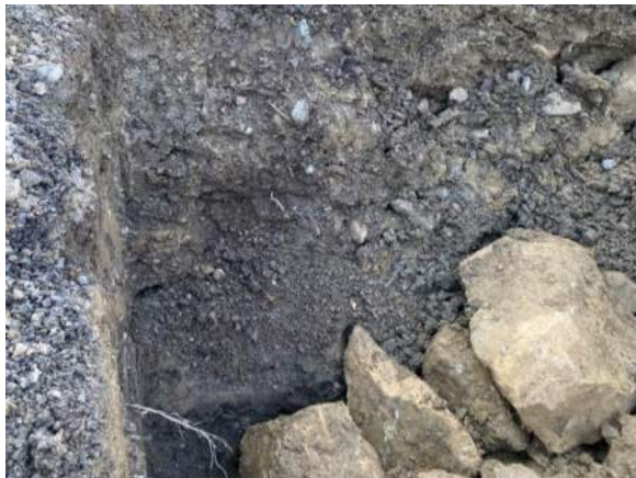
Photo #5 : TP-2, Williamstown fill soil.
