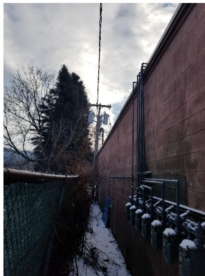
Plate 3. View is looking east along the north exterior wall.
