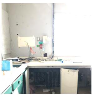
Photograph 14: View of UST system controls and location of water shutoff in Subject Property building. Veeder root fuel management system has been removed.
