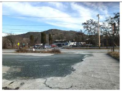
Photograph 3: Gravel portion of parkin lot is the former location of the 15,000-gallon UST. The UST was removed in 2018, backfilled with native material and surfaced with gravel. Photograph shows Main Street in background, looking northeast.
