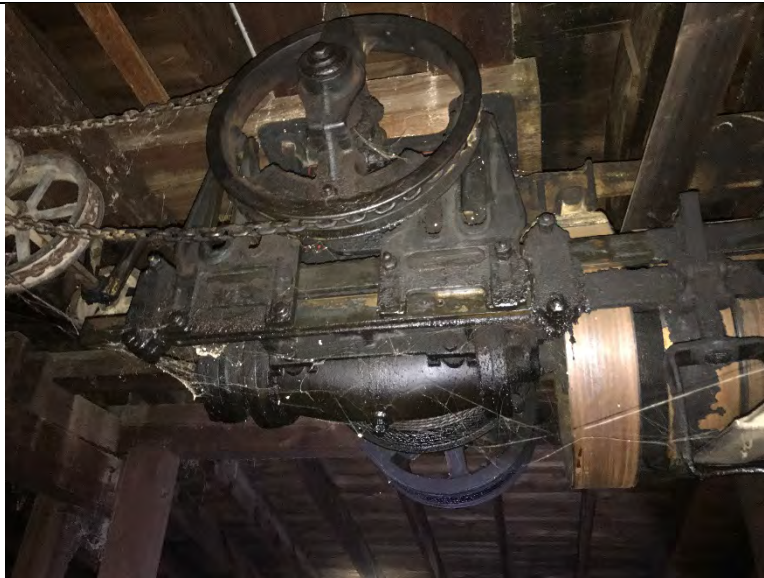
Photograph 29: Elevator pulley system located on the fifth floor of the former grain elevator and storage building.
