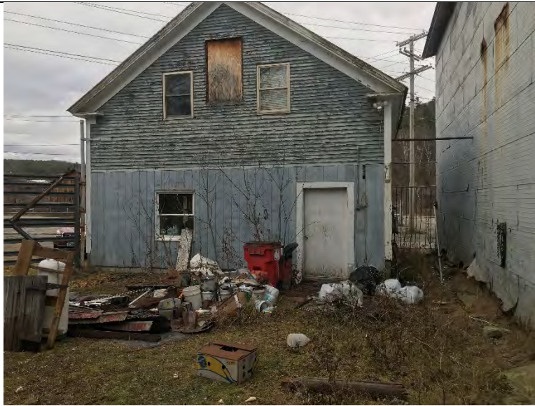
Photograph 3: Western façade of the former office building, looking east.
