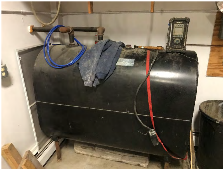
Photograph 14: 275-gallon fuel oil AST in the southern portion of the former retail and storage building.
