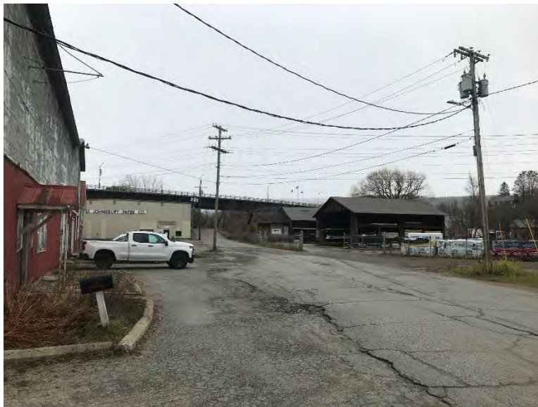
Photograph 6: Pole mounted electrical transformers east of Bay Street
