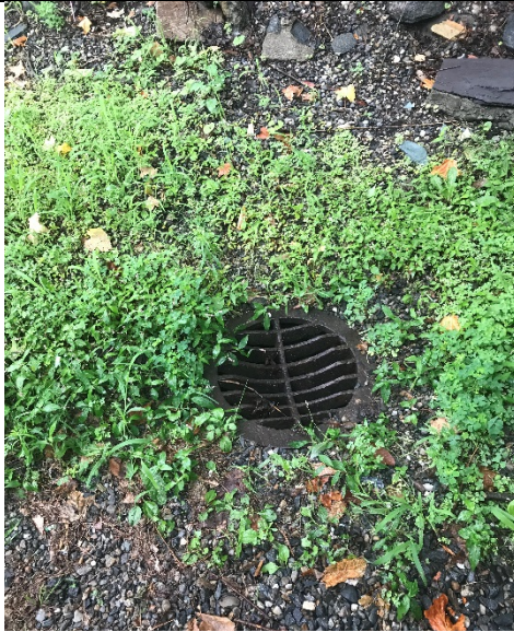
Photograph #15: Storm drain in grassy area east of building, appeared to be connected to storm system.
