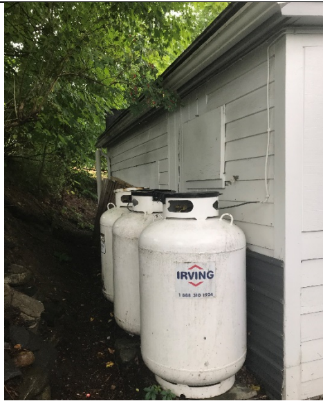
Photograph #9: Three propane tanks used as the heating fuel for the property building.
