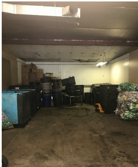
Photograph #12: Single bay garage located in southern portion of the building with overhead door.
