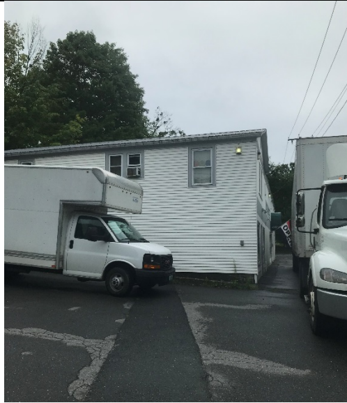
Photograph #3: View of the northern façade of Springfield Redemption Center, and second floor residential apartment, looking south from the parking area. Cut-out in pavement is the sewer line.
