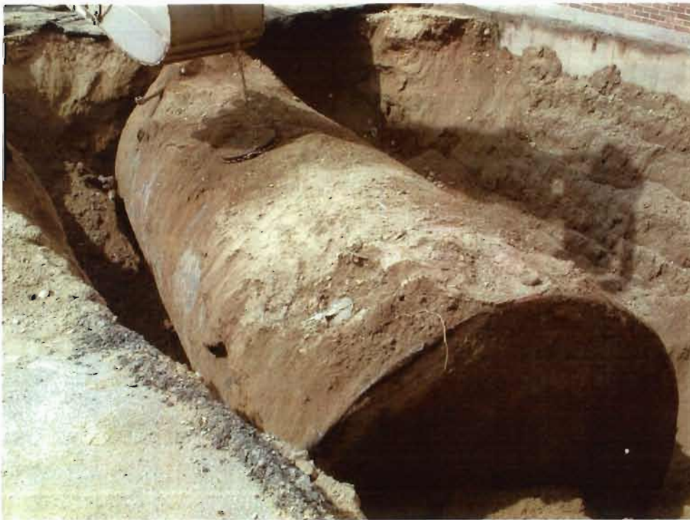
Tank being removed
