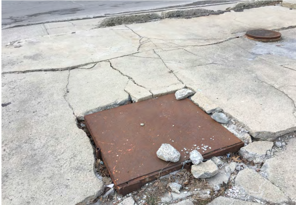
Photo 27: 25 Stebbins Street: Sewer features were observed within the concrete slab of 25 Stebbins Street. Photo taken facing northwest by Sanborn Head on January 10, 2017.
