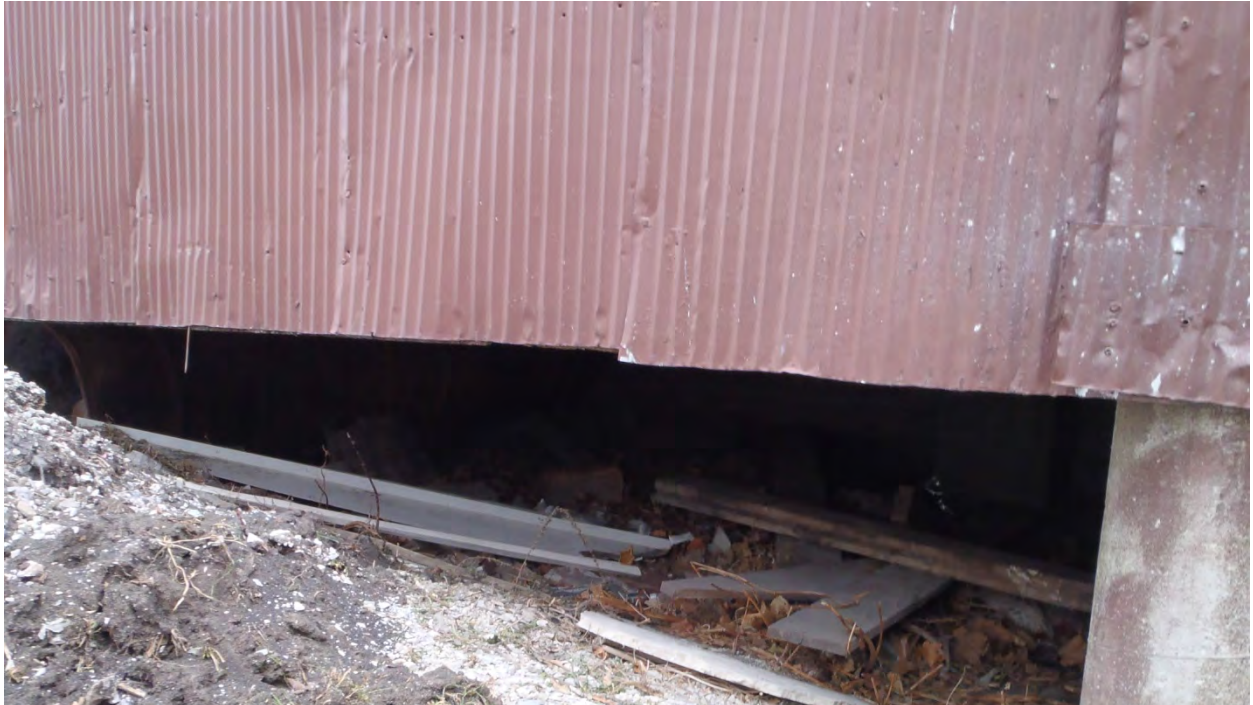
Photo 43: 23 Stebbins Street: A crawl space was observed under the former Town and Country Auto Body. Photo taken facing south by Sanborn Head on January 10, 2017.
