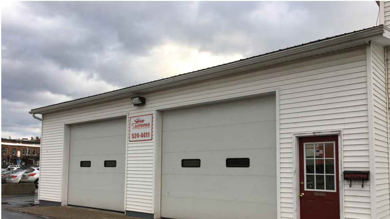
Photo 45: 13 Stebbins Street: The garage building located on the northern portion of the property is used for Auto Pro Detailing. Photo taken facing northeast by Sanborn Head on January 11, 2017.
