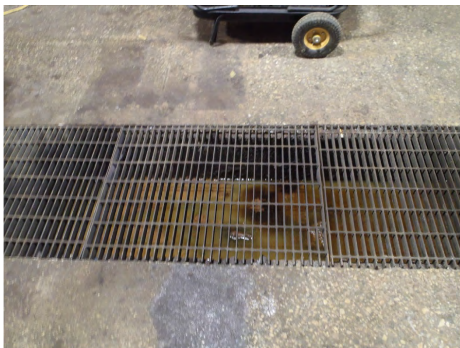
Photo 36: 21 Stebbins Street: A floor drain in the former car wash building; drain reportedly discharges to a 1,000-gallon underground grit trap in parking lot. Photo taken facing south by Sanborn Head on January 10, 2017.
