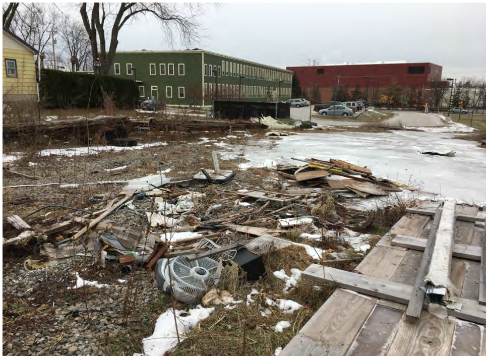
Photo 6: 14 Stebbins Street: A pile of various construction and demolition debris, as well as household items was observed behind the building located at 14 Stebbins Street. Photo taken facing southwest by Sanborn Head on January 10, 2017.
