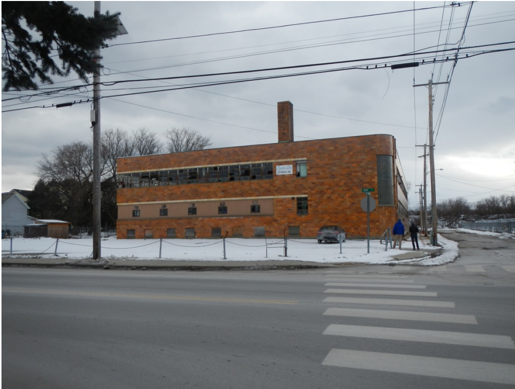
Photo 1: The Site looking south. The north side of the building, parking lot, and multiple utility poles can be seen.
