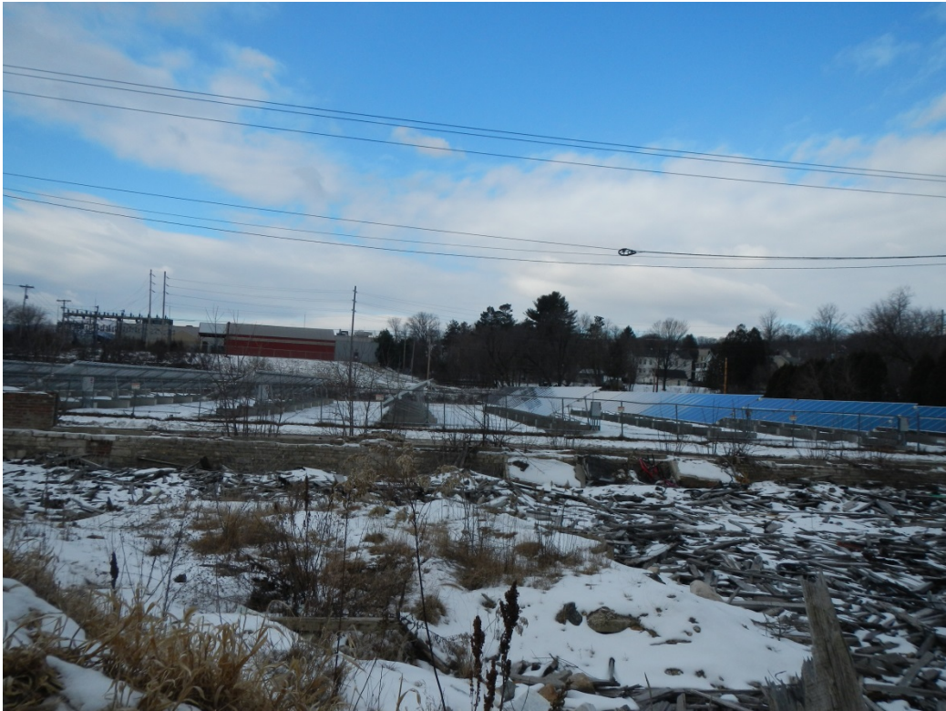
Photo 9: Photo taken looking west. Construction debris from the demolished building and the neighboring CVPS property can be seen.
