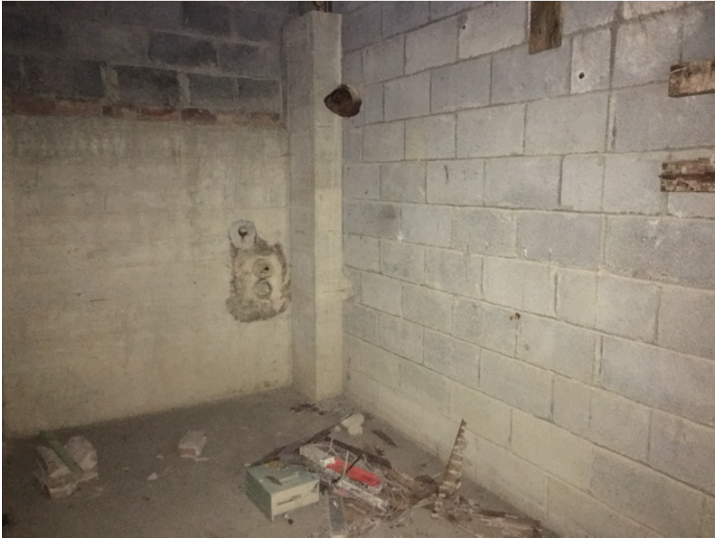
Photo 25: A room in the basement that appears to have once contained an AST located on the west side of the stairwell.
