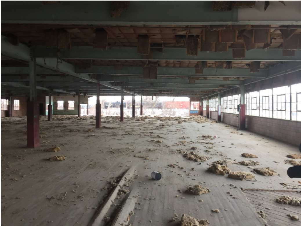
Photo 17: The top floor of the building looking south.
