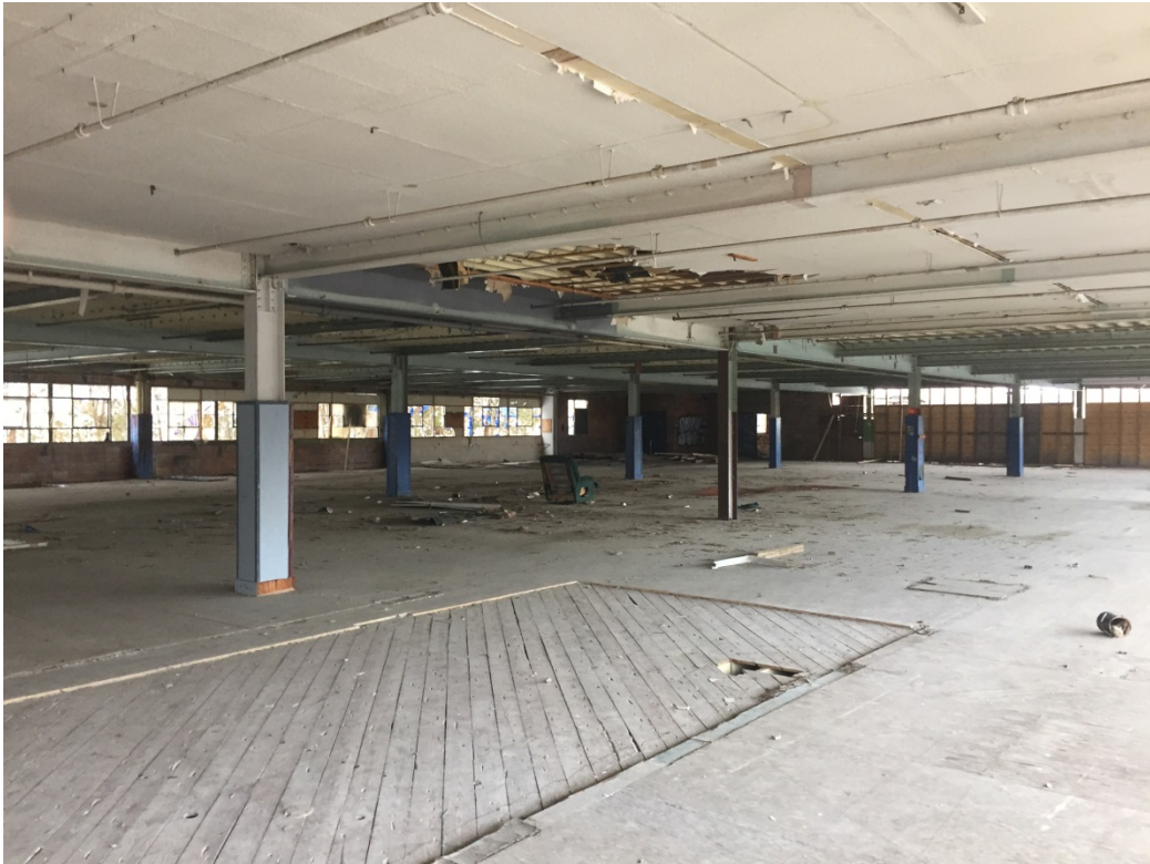
Photo 21: The first floor of the building. Photo taken looking southeast.
