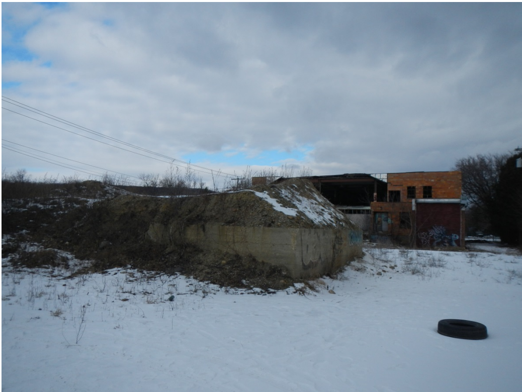
Photo 4: The south portion of the Site looking north. The fill from the stormwater construction project can be seen on the building foundation.
