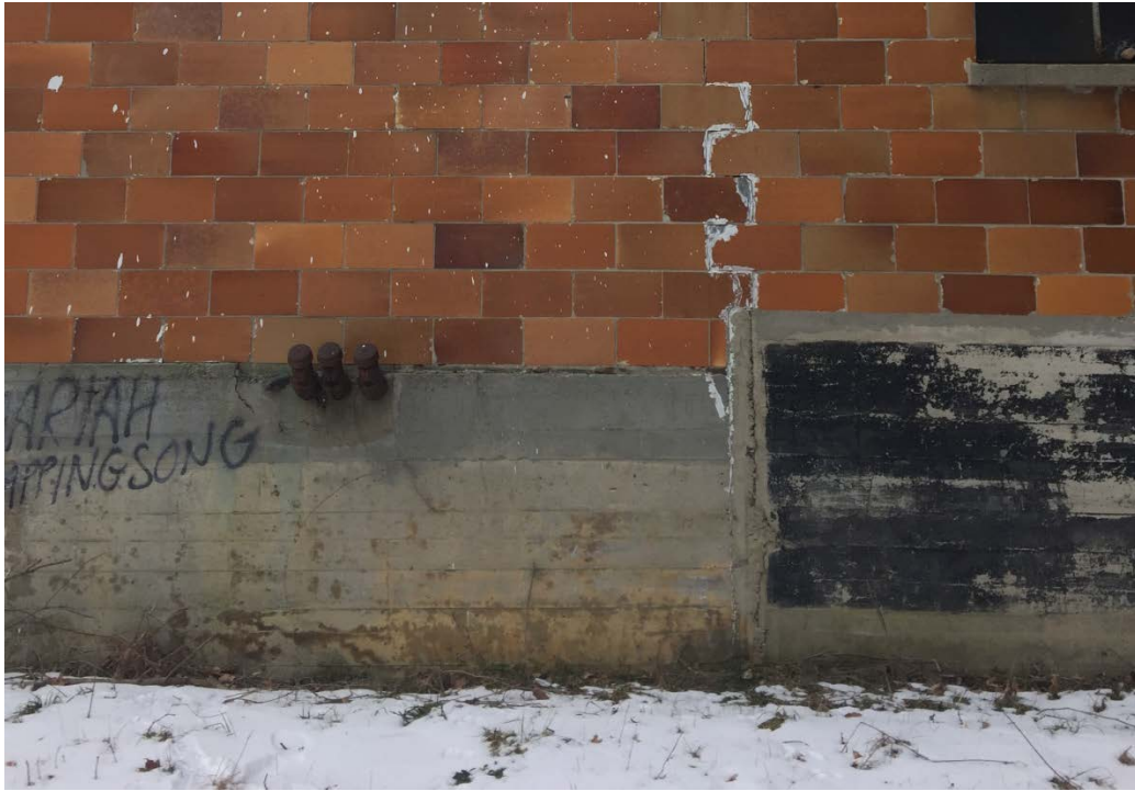
Photo 11: The three-port fill pipe and vent pipe on the east wall of the building near the southeast corner.
