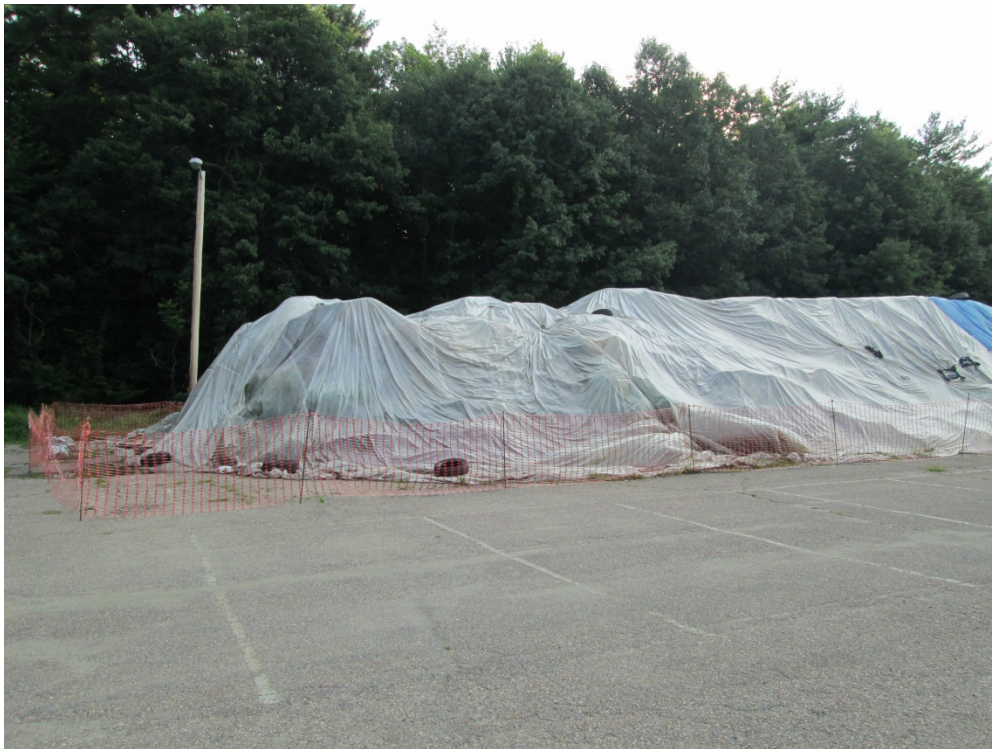
Photo 1: Soil stockpile condition before corrective action on 7/29/15. Photo taken looking east.
