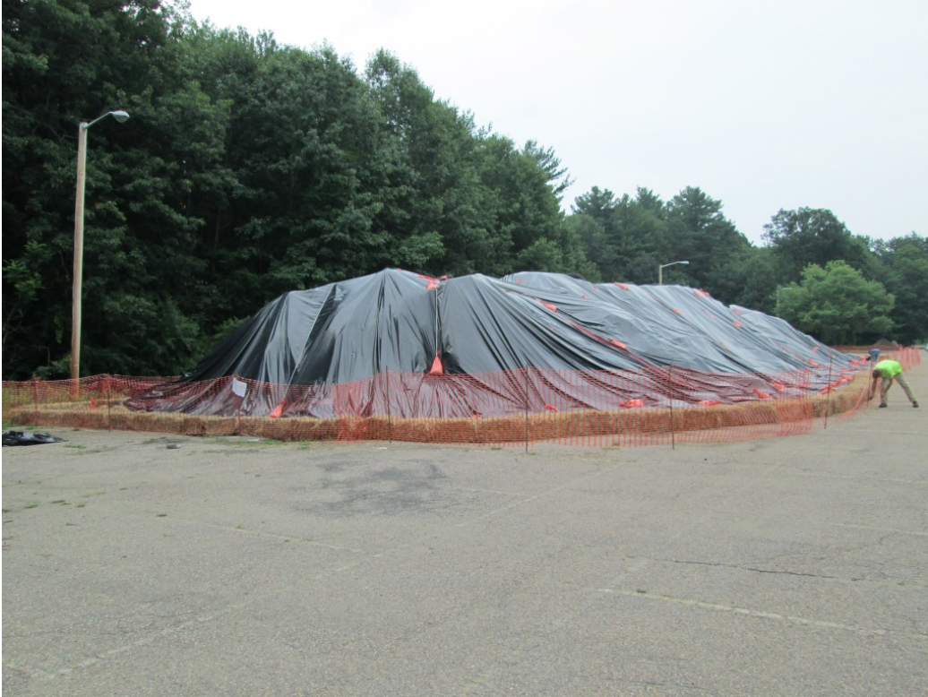
Photo 4: Soil pile after corrective action on 7/30/15. Photo taken looking southeast.
