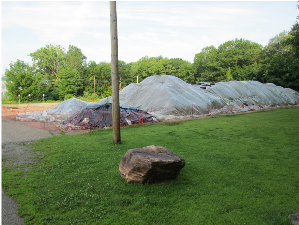
Photo 3: Soil stockpile before corrective action on 7/29/15. Photo taken looking west.
