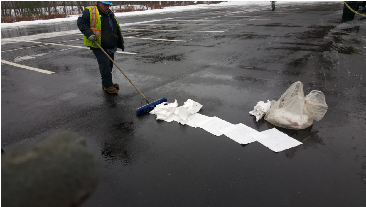
Photo 5: Collecting the sheen on the parking lot which resulted from oil drips from the dual axle dump truck
