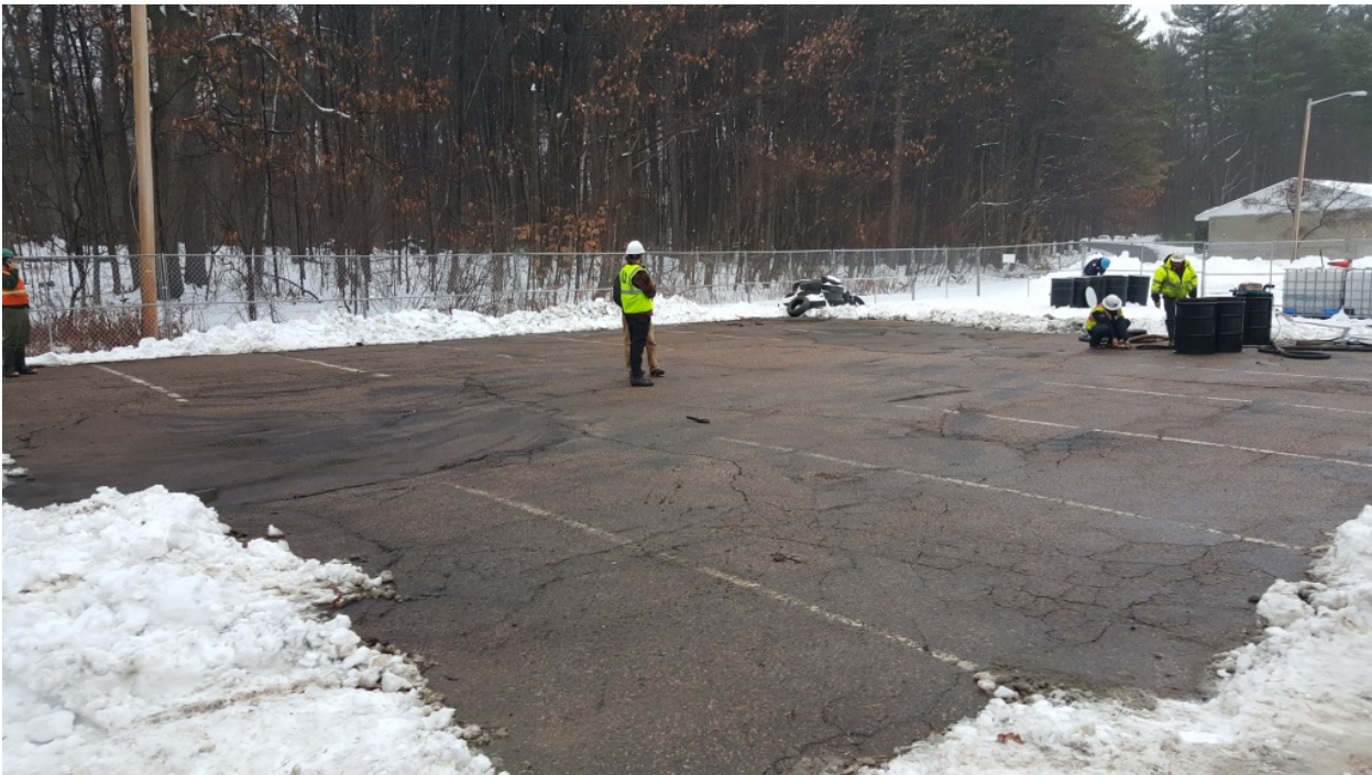
Photo 6: The parking lot condition following completion of the cleaning effort.
