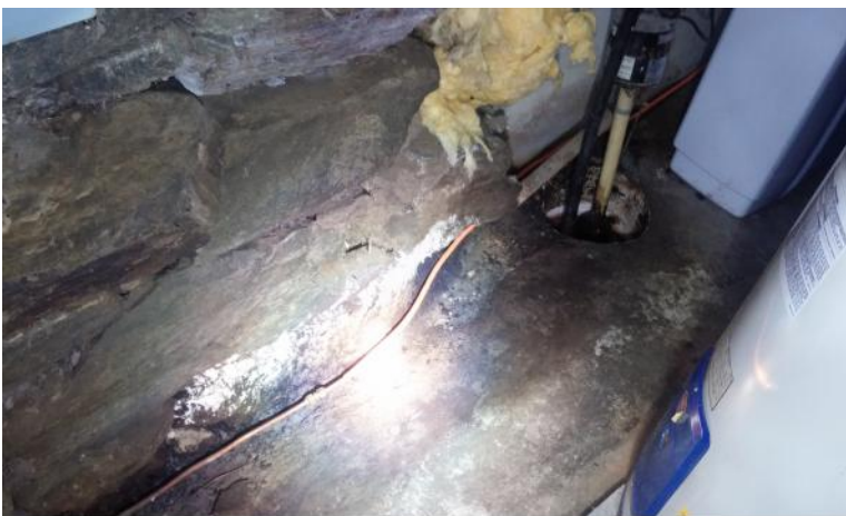
Photograph #3-Site Overview – Spill Area from Soft Copper Line.
