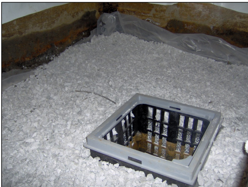
Photo #5: Sump replaced with clean gravel backfill, vapor barrier
