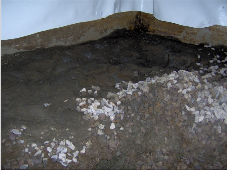
Photo #1: Sump pump removed, beginning of excavation
