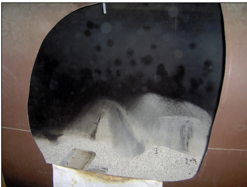
Photo #7: Fluid containerized, adsorbing remaining sludge
