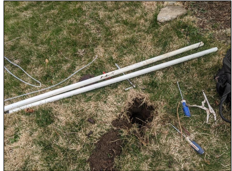
Photo #2: Well materials removed at MW-3, before backfilling.
