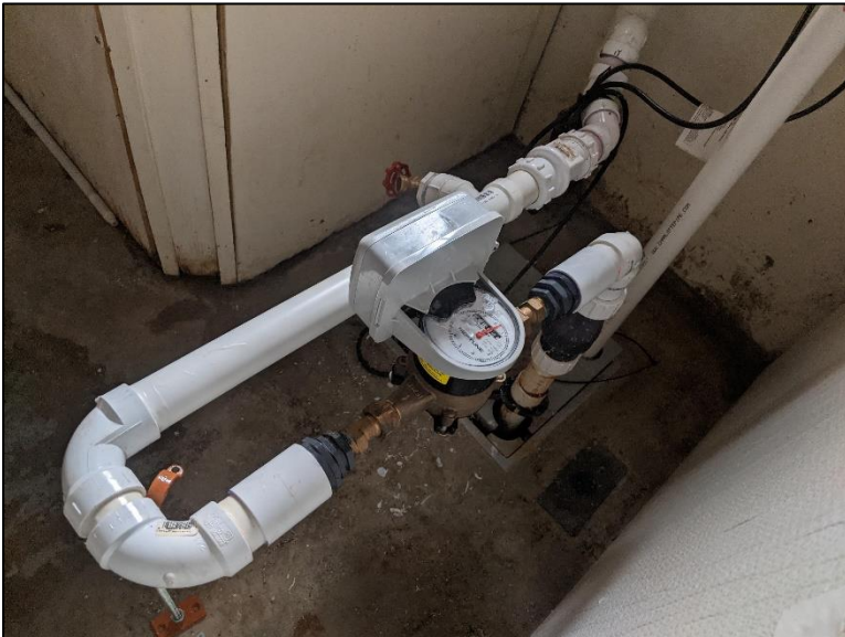
Photo #3: Totalizing flow-meter installed in-line with 1.5" PVC.
