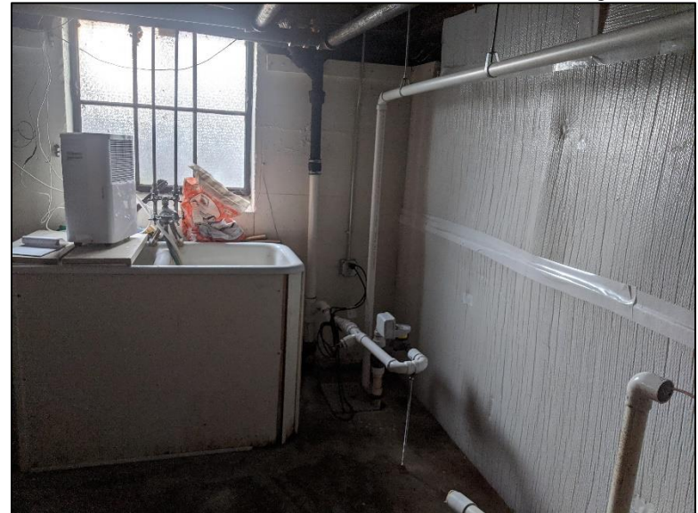
Photo #4: Full system restored, showing connection to sanitary sewer (black pipe)
