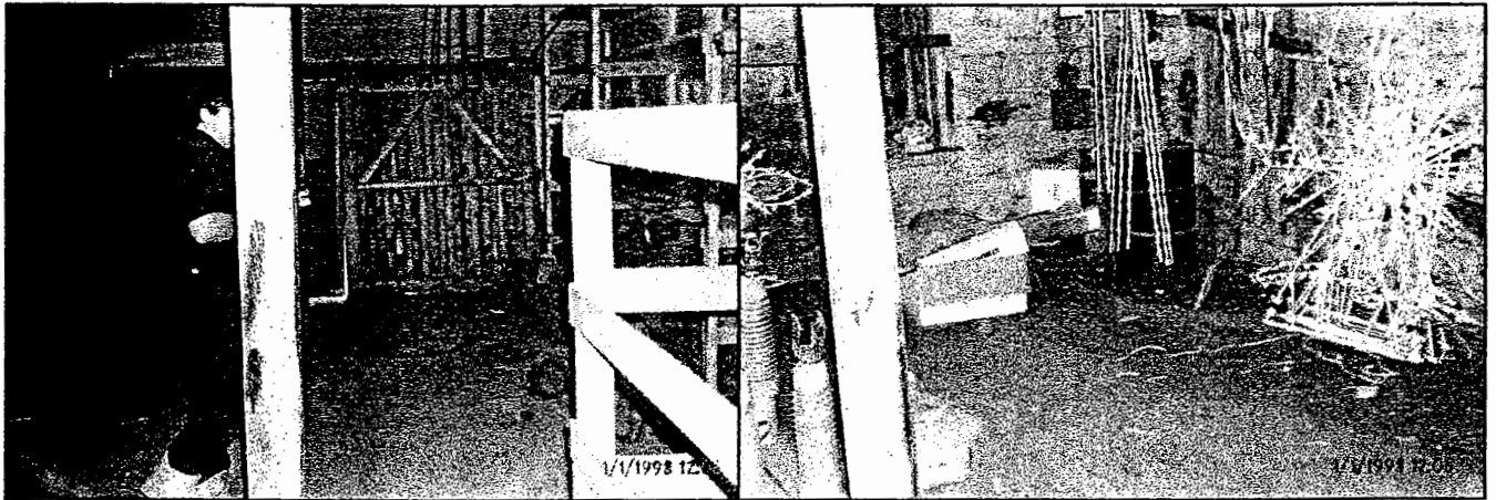
Photographs 13 & 14: Contents of Building No. 2 2 nd floor. Buidling No. 2 3 rd floor.
