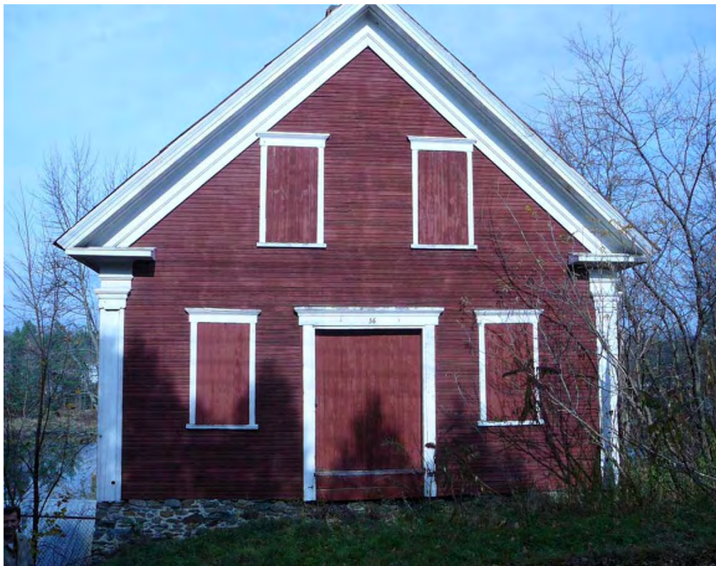
Figure 8. View northwest of front façade of the creamery from A Street, Morrisville, Vermont.
