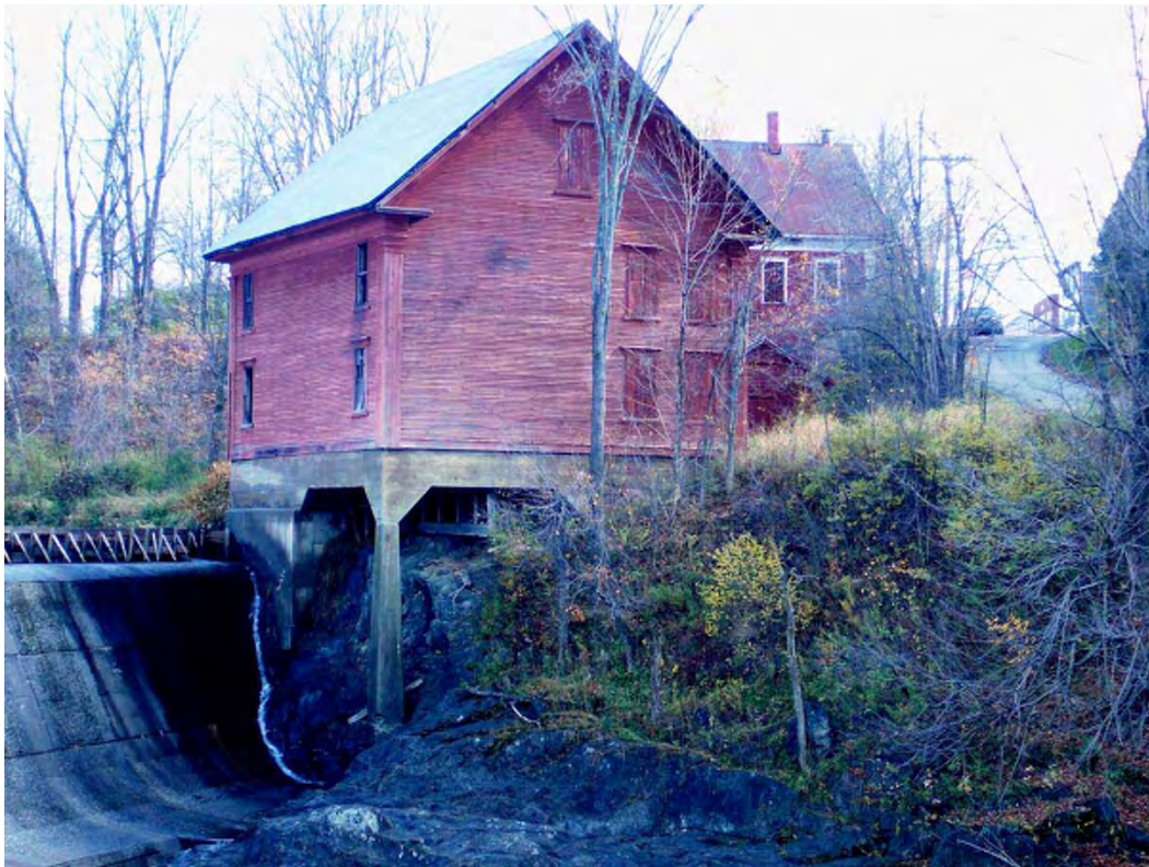
Figure 5. View northeast of the grist mill with creamery in background, Morrisville, Vermont.
