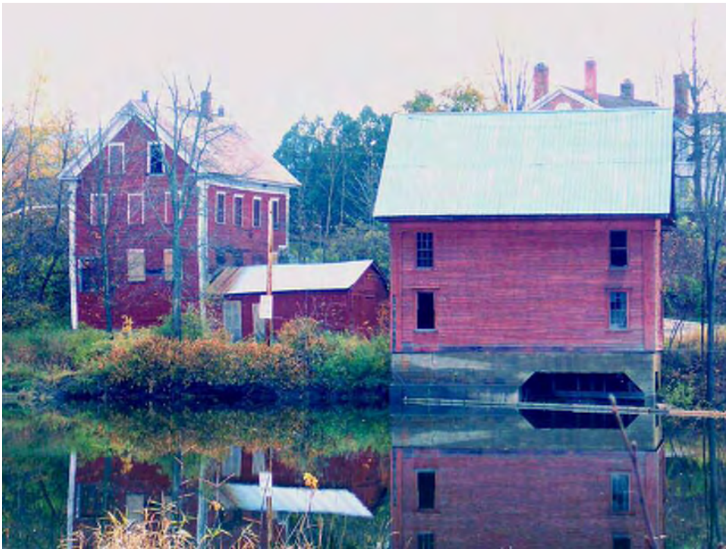
Figure 3. View northeast of the grist mill (right) and creamery (left) buildings along the Lamoille River, in Morrisville, Vermont.
