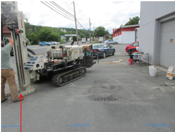
Looking easterly, drilling SB3
