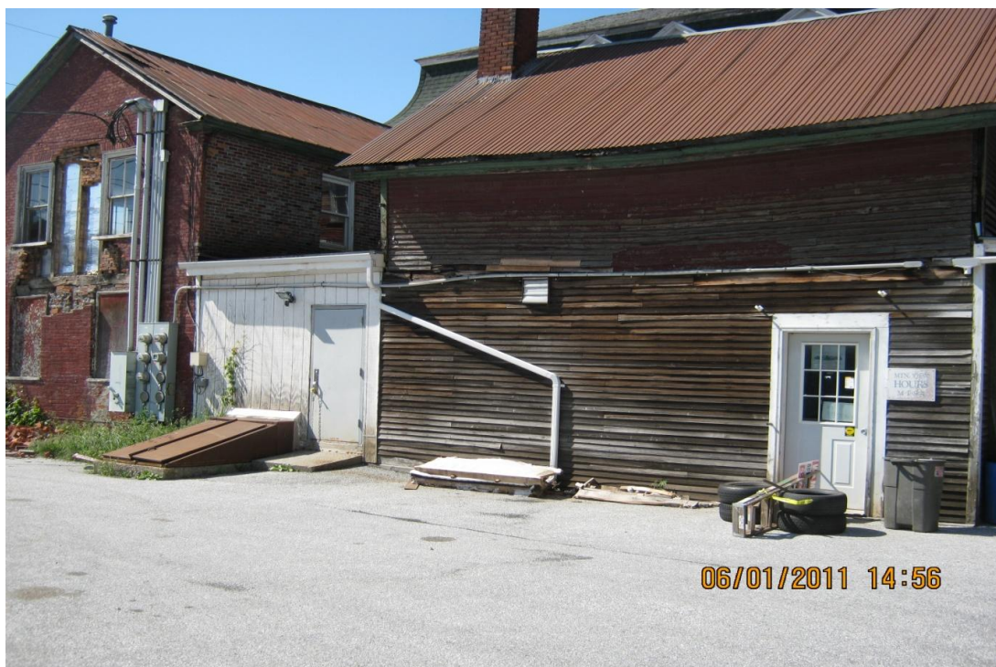
Rear of outbuildings at site, facing north
