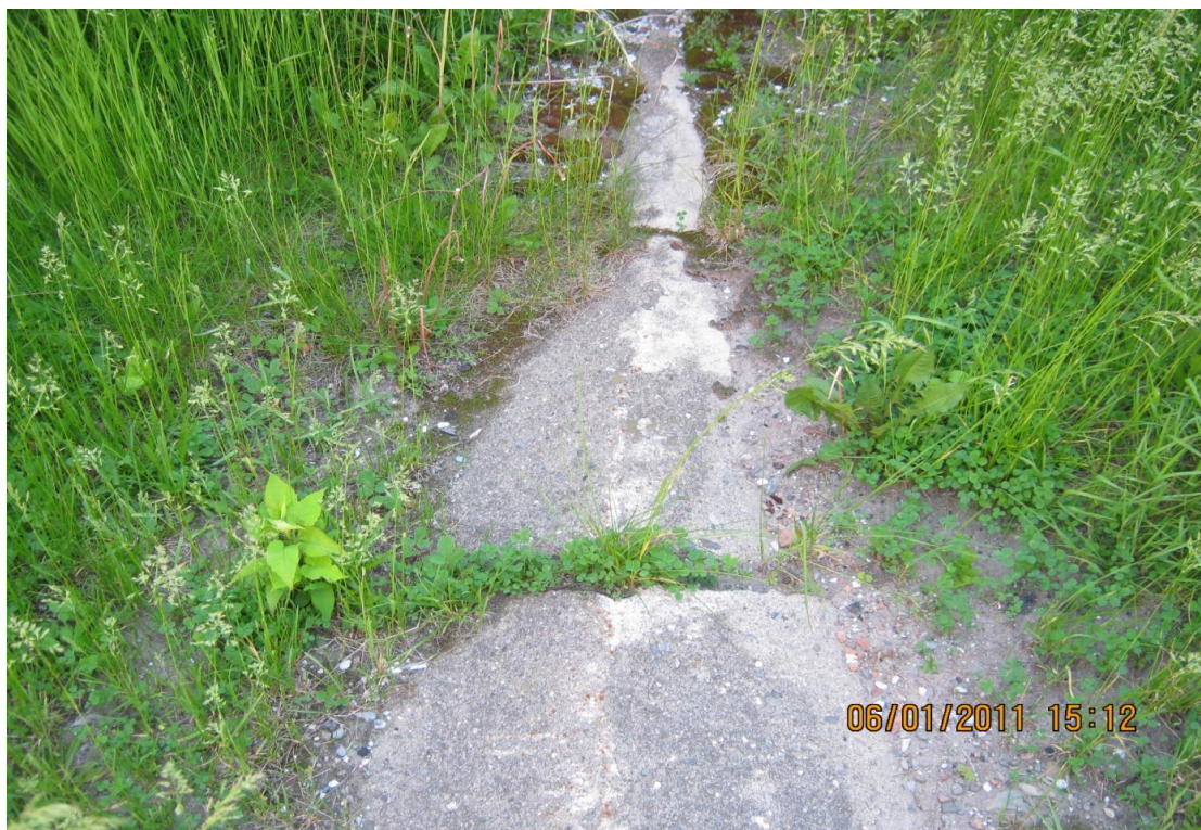
Unidentified concrete structure outside of east side of building
