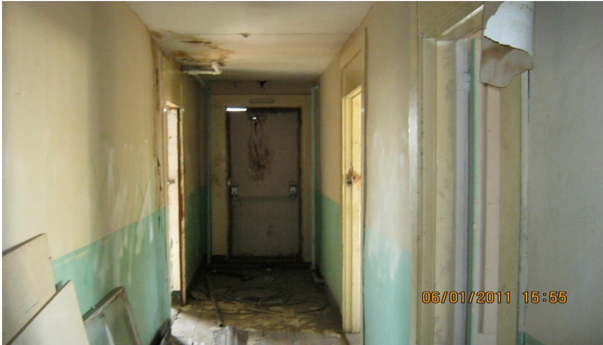
Typical tenant room hallways on 2 nd , 3 rd , and 4 th floors
