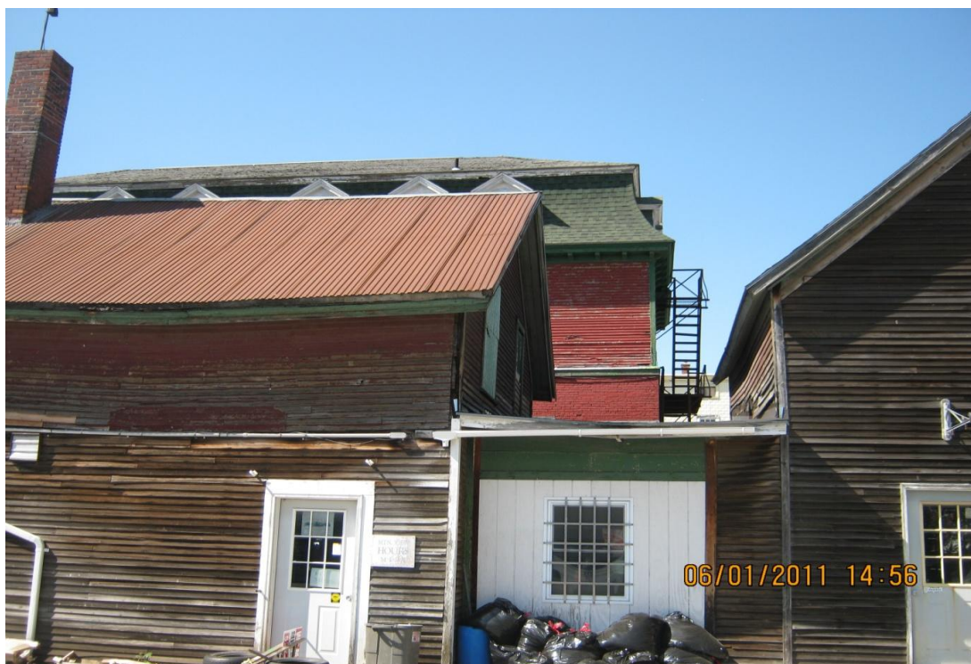
Rear of outbuildings at site with main 4-story structure in background, facing north
